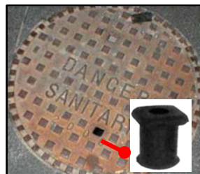
Sealing Sanitary Manhole Covers in Low Lying Areas
