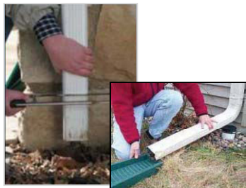
Downspout Disconnection
