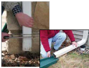
Downspout Disconnection
