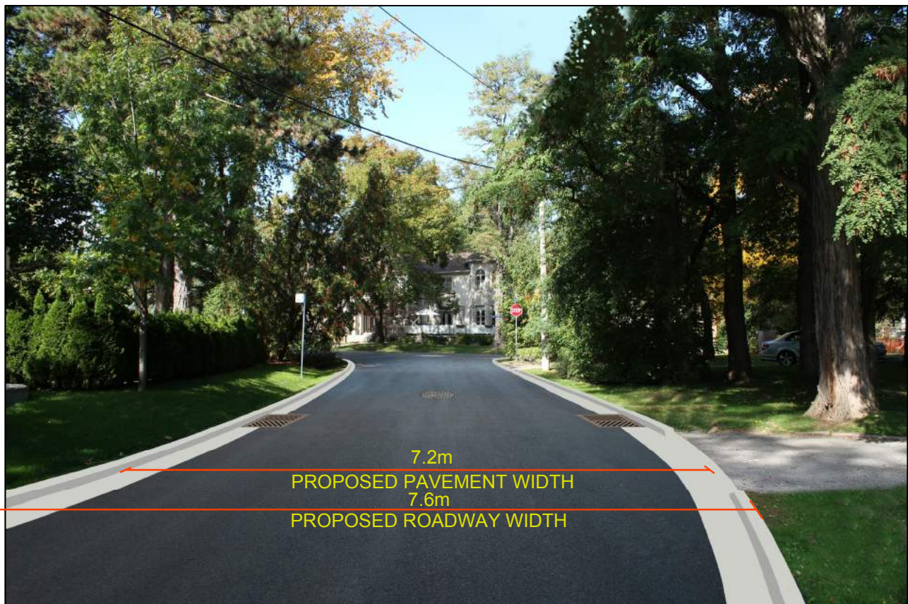
FIGURE LE2 ILLUSTRATION OF EXISTING AND PROPOSED ROAD DIMENSIONS - LEWES CRES
