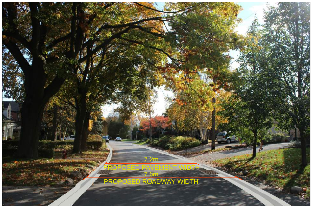
FIGURE MN1 ILLUSTRATION OF EXISTING AND PROPOSED ROAD DIMENSIONS - MILDENHALL RD (NORTH OF LAWRENCE AVE E)
