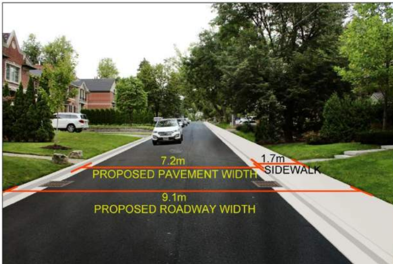
FIGURE SL1 ILLUSTRATION OF EXISTING AND PROPOSED ROAD DIMENSIONS - ST LEONARDS AVE
