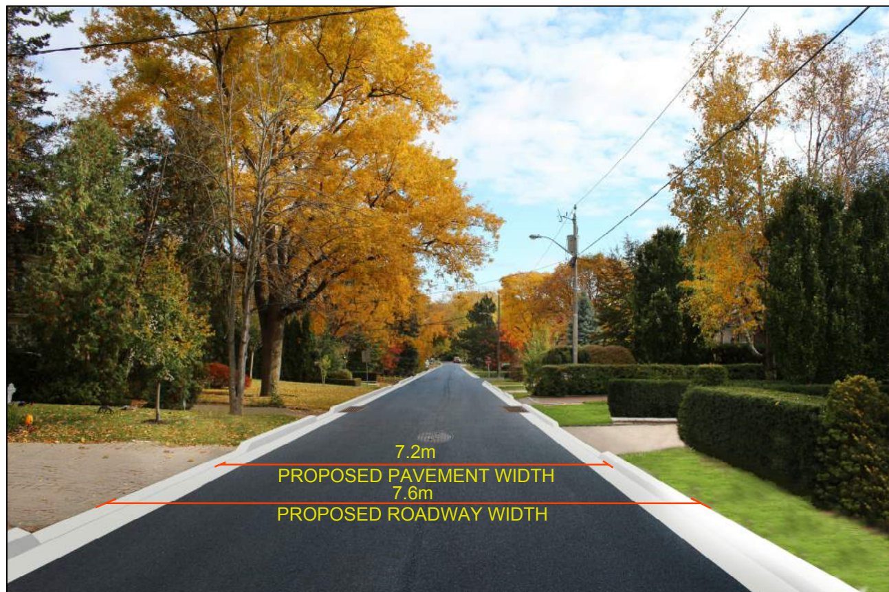
FIGURE RO1 ILLUSTRATION OF EXISTING AND PROPOSED ROAD DIMENSIONS - ROCHESTER AVE
