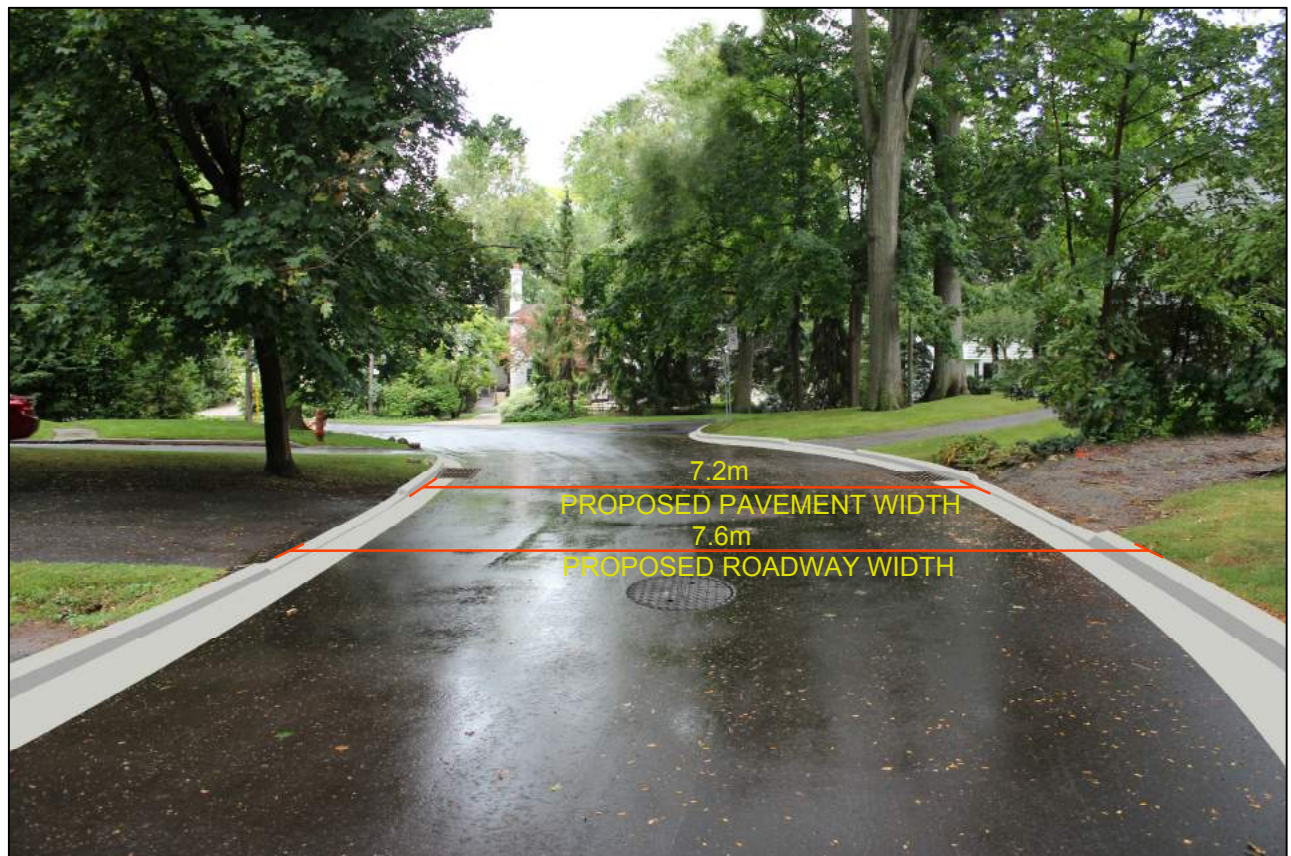
FIGURE BW3 ILLUSTRATION OF EXISTING AND PROPOSED ROAD DIMENSIONS - ST AUBYNS CRESCENT
