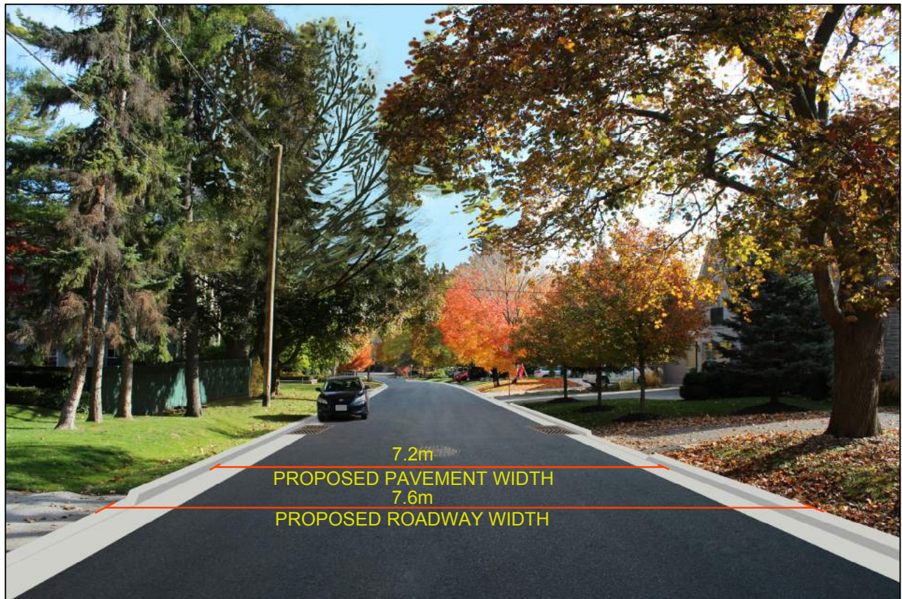
FIGURE RM1 ILLUSTRATION OF EXISTING AND PROPOSED ROAD DIMENSIONS - ROTHMERE DR
