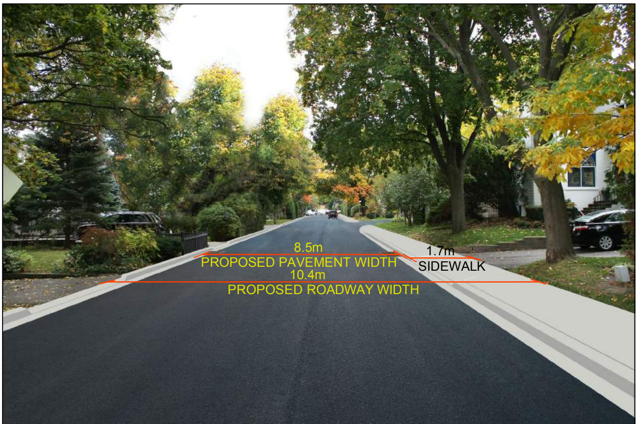
FIGURE ML5-1SW ILLUSTRATION OF EXISTING AND PROPOSED ROAD DIMENSIONS - MILDENHALL ROAD SOUTH OF CHELTENHAM AVE
