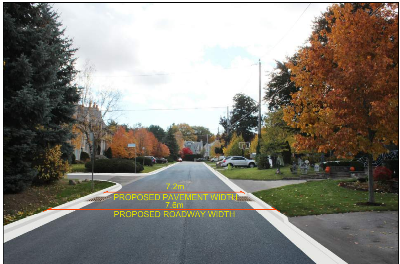
FIGURE BH1 ILLUSTRATION OF EXISTING AND PROPOSED ROAD DIMENSIONS - BLYTH HILL RD
