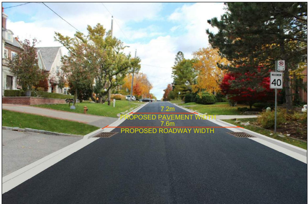
FIGURE SD1 ILLUSTRATION OF EXISTING AND PROPOSED ROAD DIMENSIONS - STRATHEDEN RD
