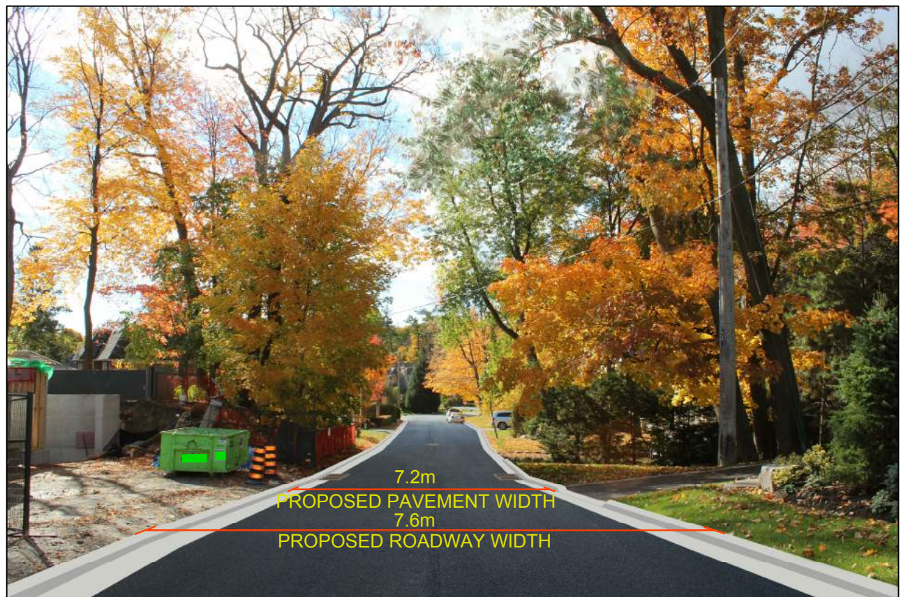
FIGURE FI1 ILLUSTRATION OF EXISTING AND PROPOSED ROAD DIMENSIONS - FIDELIA AVE
