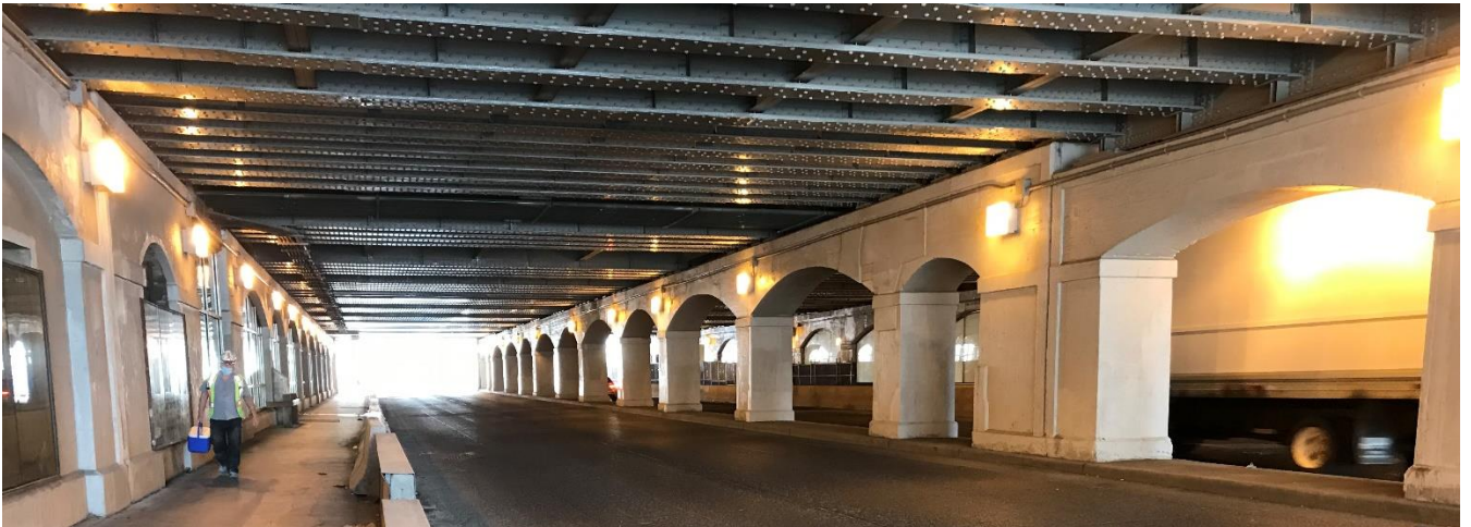
Plate 73: North-northwest view of Bay Street showing centre row of columns supporting the Union Station Trainshed. All columns will be retained and supported with new infrastructure below grade.
