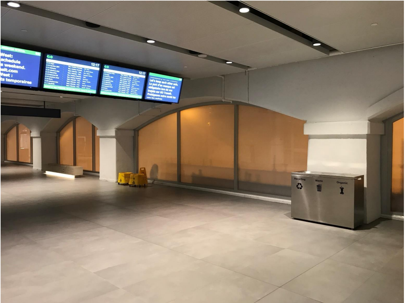
Plate 83: Interior of the East Teamway showing columns and segmentally arched openings in good repair. The columns and arches have been coated in white protective sealer and the glass panes have been replaced.
