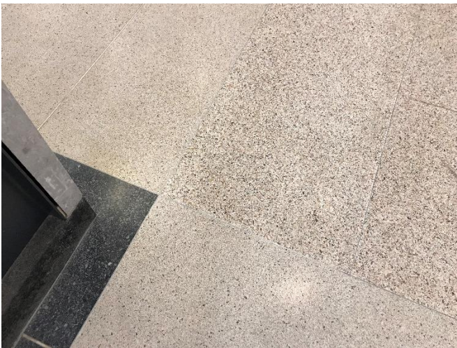
Plate 35: Terrazzo flooring in the concourse level of the east block
