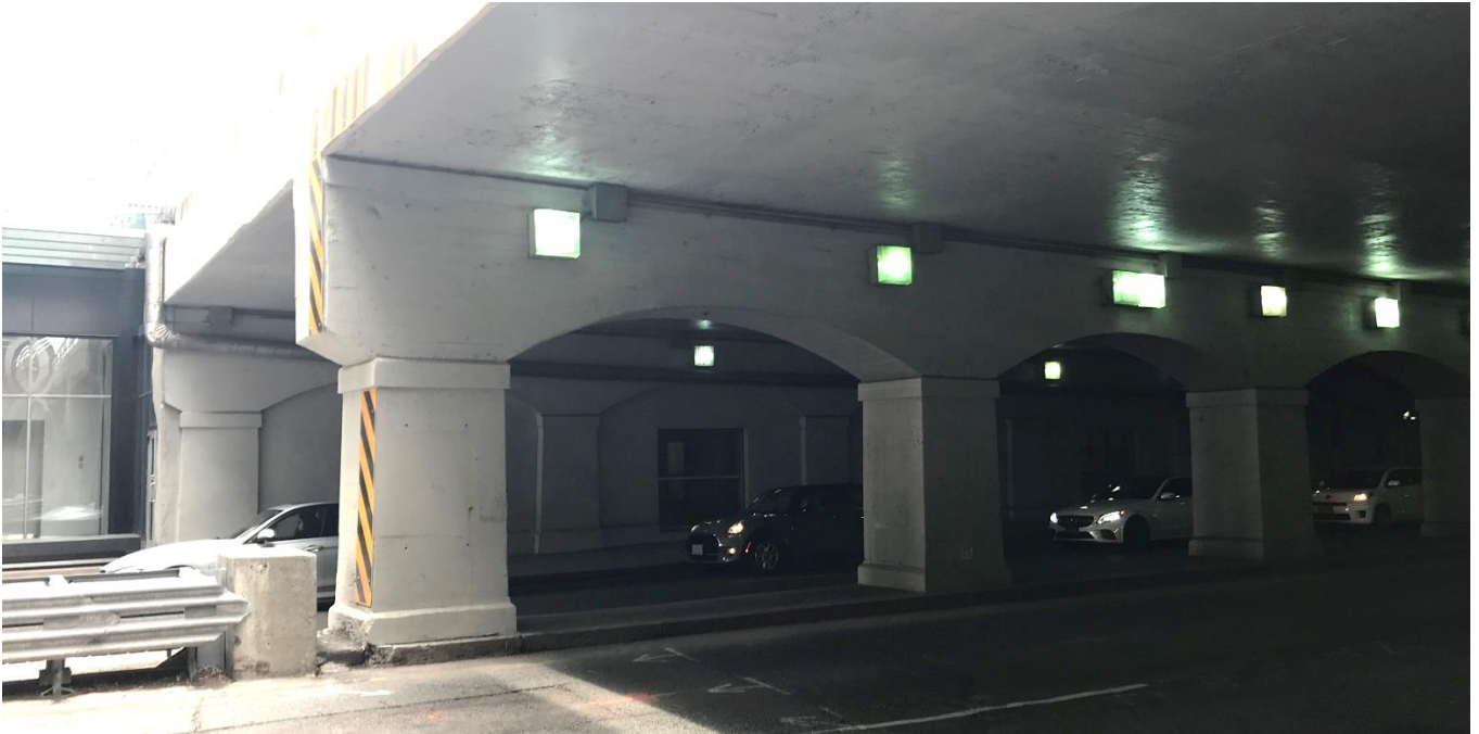
Plate 84: Photo of the central columns and segmentally arched openings on York Street. The columns located in the median along York Street appear to be in good repair and have been coated in a light grey protective sealer.
