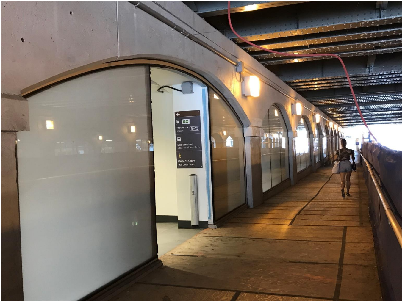
Plate 82: Exterior of the concrete columns with segmentally arched openings on the east side of Bay Street (leading to the East Teamway). The columns on the east side of Bay Street are in good repair and have been coated in light grey protective sealer
