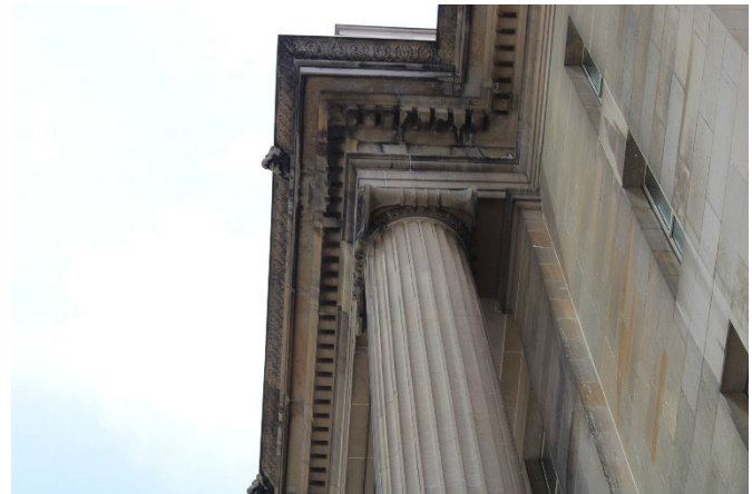
Plate 41: Close-up view of freestanding ionic column and dentils on the north elevation
