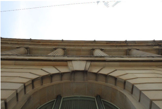
Plate 40: Close-up view of freestanding ionic columns and keystone on the north elevation
