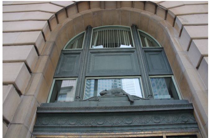
Plate 33: Metal mullions with rope detailing located above the first-storey entrance
