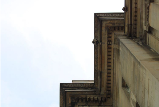
Plate 42: Close-up view of Dentil trim located on the north elevation
