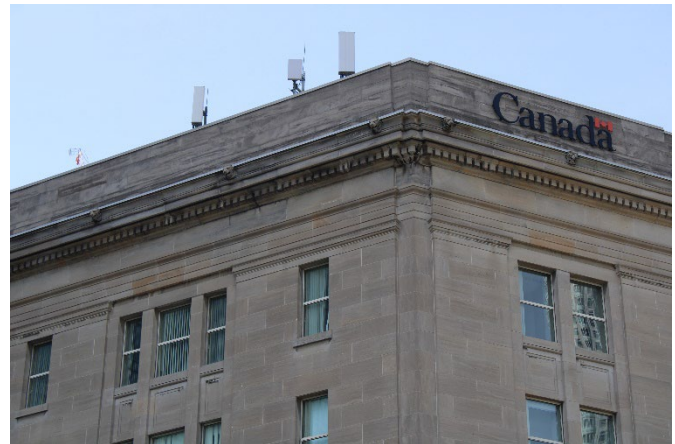
Plate 55: Upper Cornice and dentil detailing with 'Canada' sign located on the northeast corner of the building
