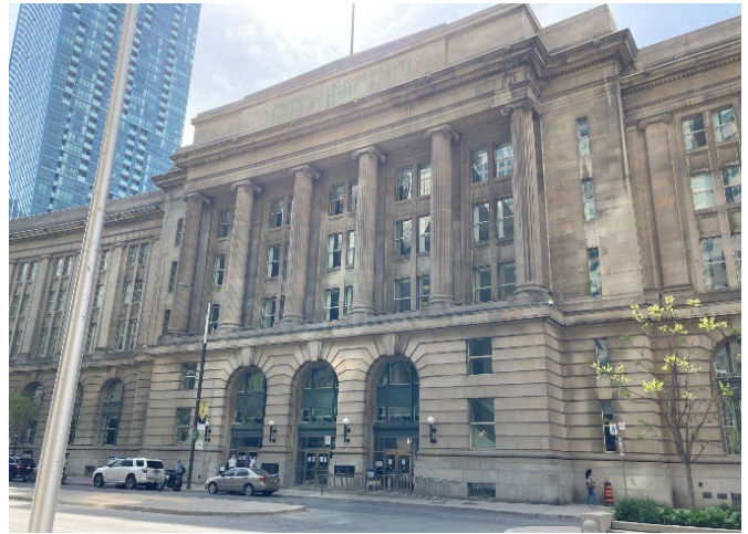
Plate 37: Central pavillion including the projecting extension, freestanding ionic columns and inscribed entablature
