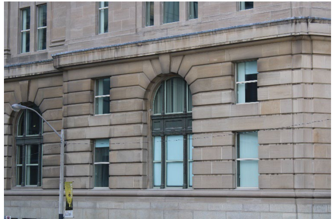
Plate 49: Example of a first-storey window on the east elevation featuring metal mullions incorporating rope detailing
