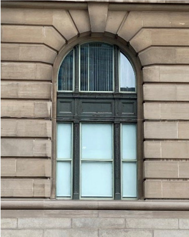
Plate 50: Example of a first-storey window on the west elevation featuring metal mullions incorporating rope detailing
