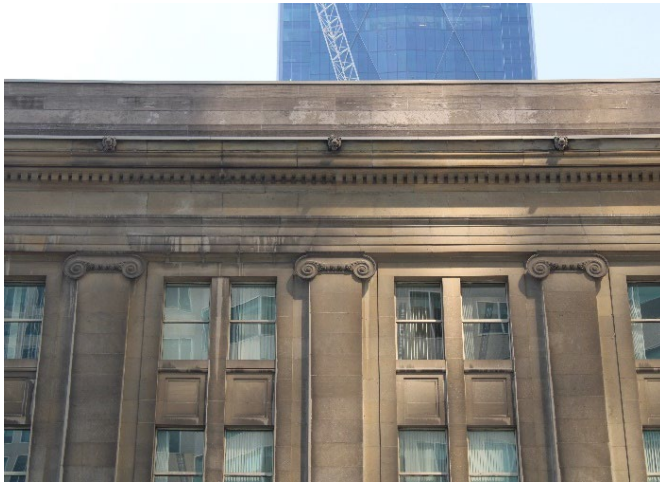
Plate 36: Upper cornices with the dentils, engaged ionic columns and stone lion's heads.
