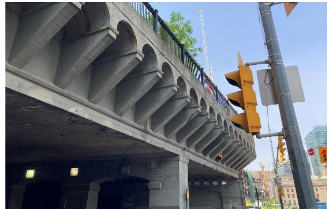
Plate 19: View of the projecting beams with decorative semi-circular arches at the beam ends on the north elevation of the Yonge Street Railway Bridge
