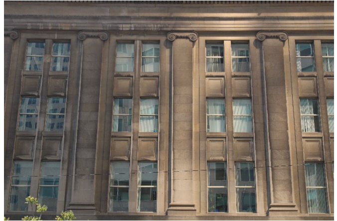
Plate 35: Engaged ionic columns on the north elevation
