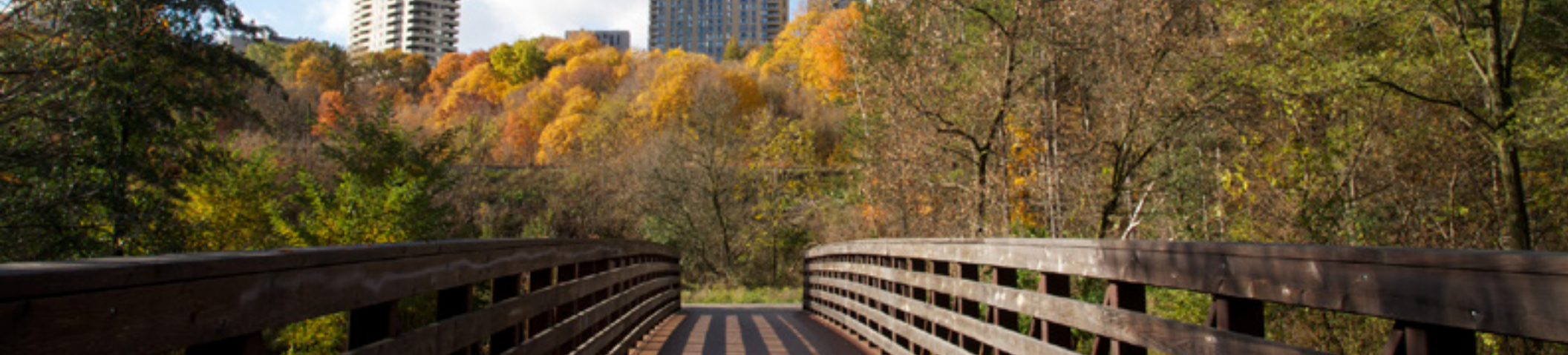
City of Toronto, Footbridge over the Don River
