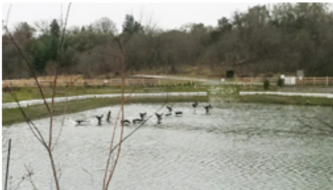
Photo: The Emery Creek stormwater ponds and wetland project will improve water quality while adding greenery and recreation space for the community. The wetland provides habitat and removes solids, and the finishing pond (right) provides final treatment before discharge to the Humber River.
