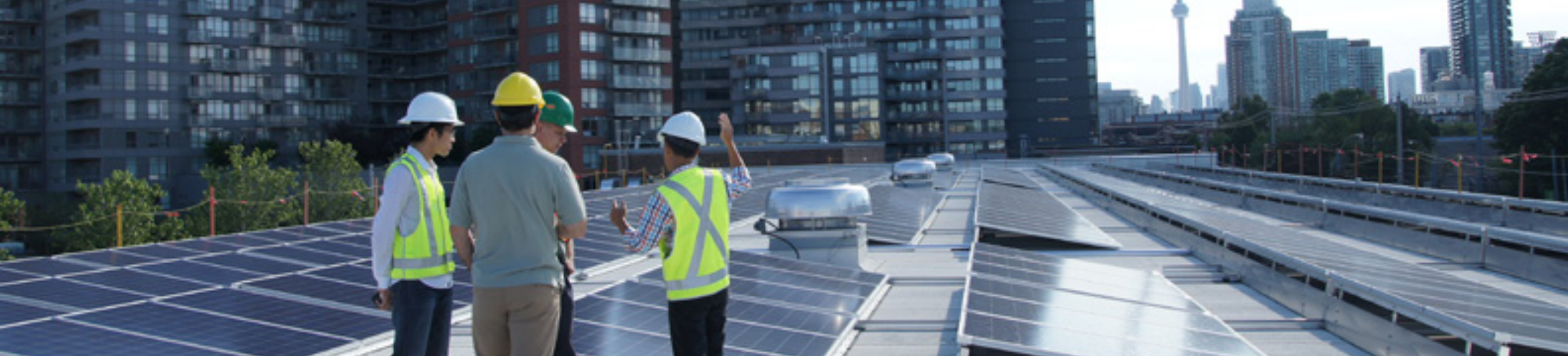
Photo: Solar PVs are installed at the City's King Street Yard (King Street W. near Dufferin Street).
