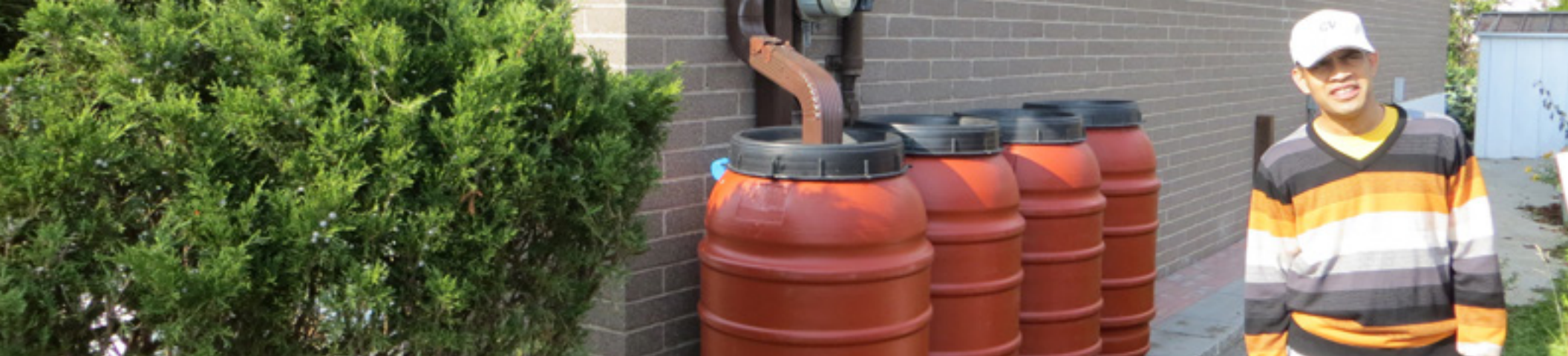
In addition to energy and basement flooding prevention retrofits, many residents in the Black Creek SNAP have installed multiple barrels to harvest the rain for their vegetable gardens.
