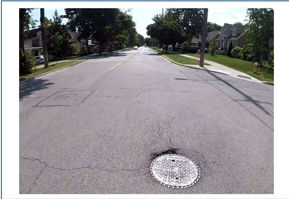
Photograph 1-3 — Martin Grove Road, about 10 m north from Donalbert Road, looking south, showing low to medium severity longitudinal and transverse cracking and low severity utility patching [28/08/2020, SG].
