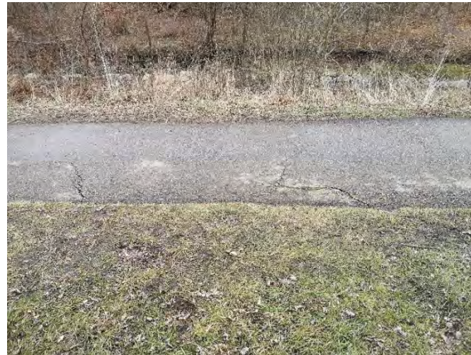
Image 4: View of field conditions during the property inspection. Note the asphalt pathway and channelled Mimico Creek.
