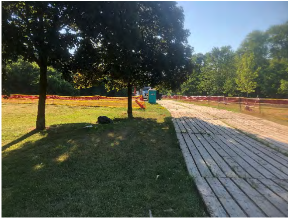
Photo 1: View of 2020 construction activity in Ravenscrest Park near Breeding Bird Station 1.
