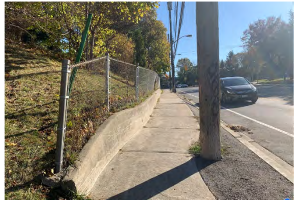
Photo 15: View facing south along the north side of Martin Grove Road, on the south side of the Mimico Creek Valley (section to be tunneled), November 4, 2020.
