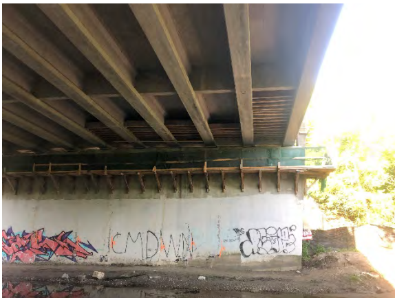
Photo 3: 2020 Bridge Repairs at Rathburn Bridge.
