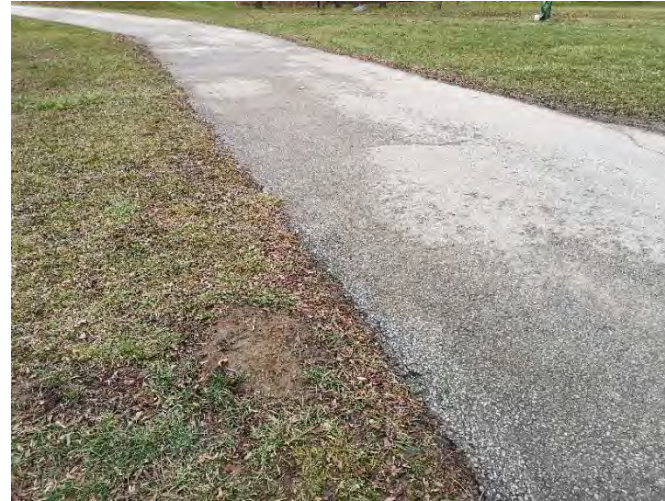
Image 2: View of field conditions during the property inspection. Note the presence of the asphalt pathway.
