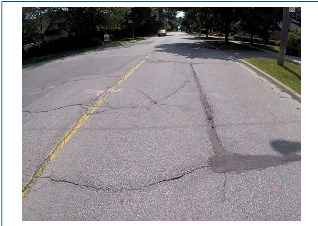
Photograph 1-4 — Martin Grove Road, about 20 m north from Lorraine Gardens, looking south, showing low to medium severity longitudinal and transverse cracking, low severity alligator cracking, low severity patching and low to medium severity depression [28/08/2020, SG].
