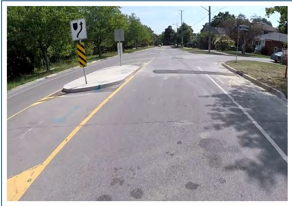
Photograph 1-1 — Martin Grove Road, about 30 m north of Saralou Court, looking south, showing low severity transverse cracking and low severity patching [28/08/2020, SG].
