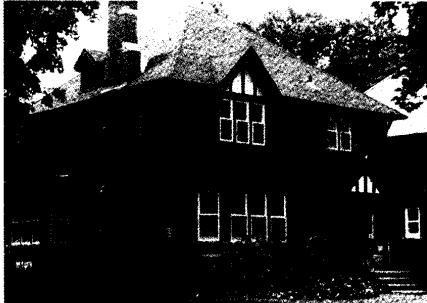
Built in 1933, this corner house is constructed mostly of tapestry brick and trimmed with small sections of stone, stucco and half timbering.
