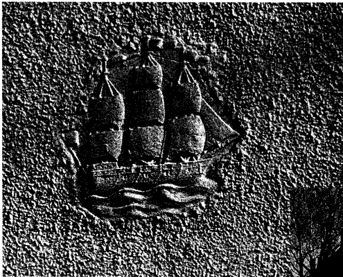
Some exterior walls contain unique features.
