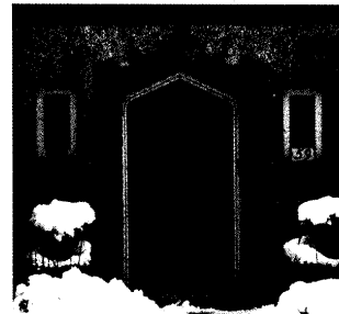
Gothic entrance with plank door and ornamental wrought-iron straps framed in stone.
