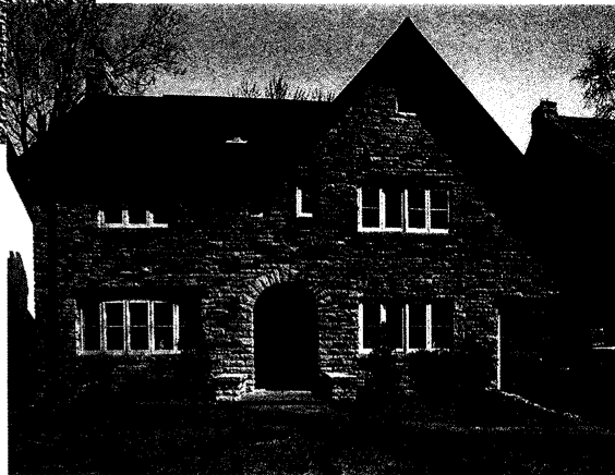
"Found stone" was used on a limited number of the earlier homes in the Park.
