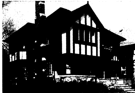
The east facing main floor bay windows now include overhanging gables of stucco and timber...a larger two storey section of matching brick and stucco-timber was added on the northeast side.
