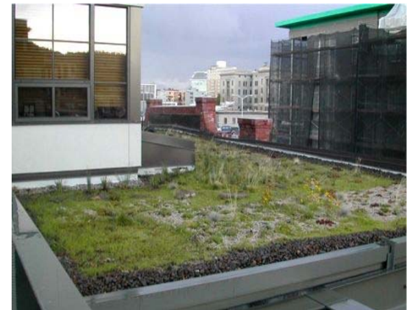
Ecotrust's John Vollum Natural Capital Centre Photo courtesy of Linda S. Velazquez
