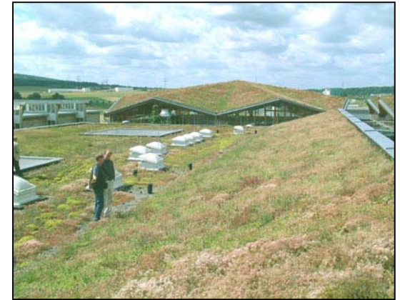
A sloped green roof on a commercial building in Kassel, Germany. Photo courtesy of Brad Rowe
