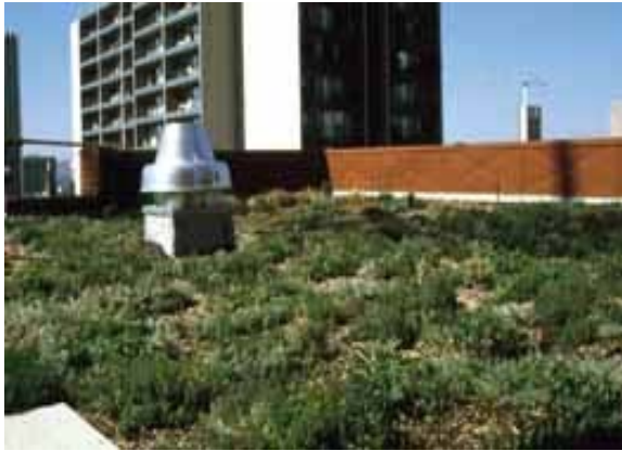
Hamilton Building in Portland Source: Green Roofs for Healthy Cities www.greenroofs.org
