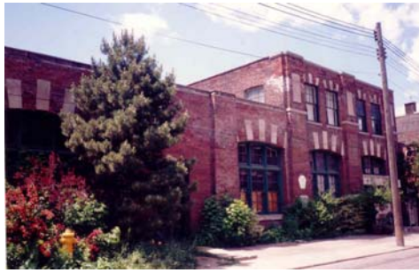
south of courtyard
