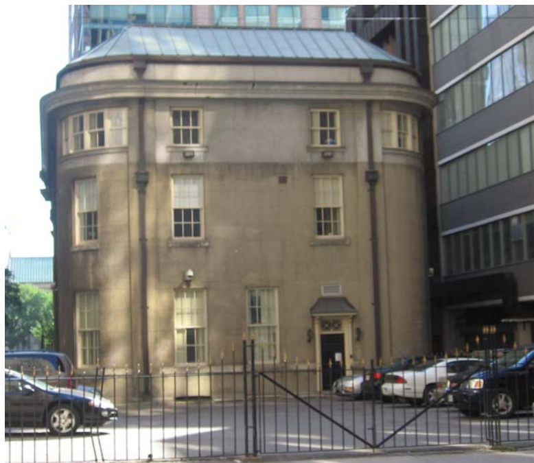
rear (west) wall
