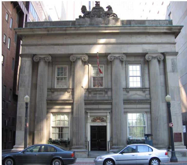
principal (east) facade
