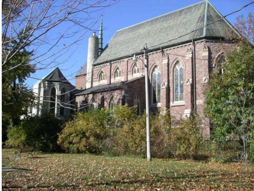
100 Howland Avenue – St. Alban the Martyr Church, looking north
