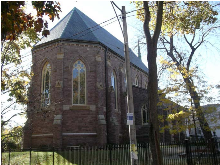
100 Howland Avenue – St. Alban the Martyr Church, looking south-west
