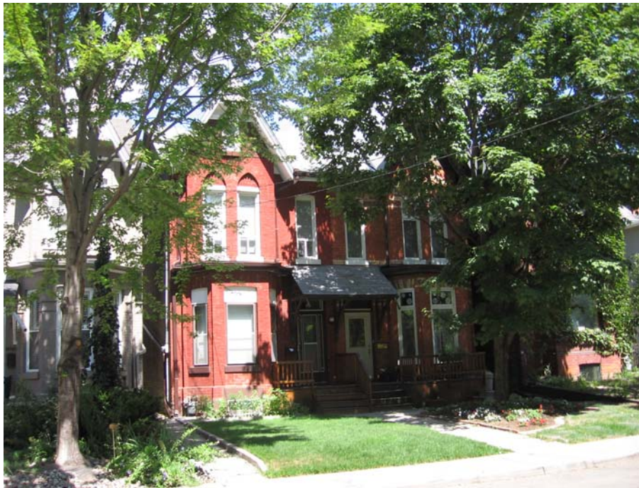
#40-42 Russell with pointed-arch window openings (left) and pattern brick detailing (right)
