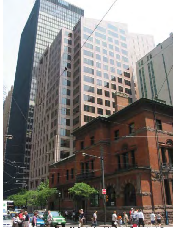
Figure 32. South side of Wellington Street at York Street
