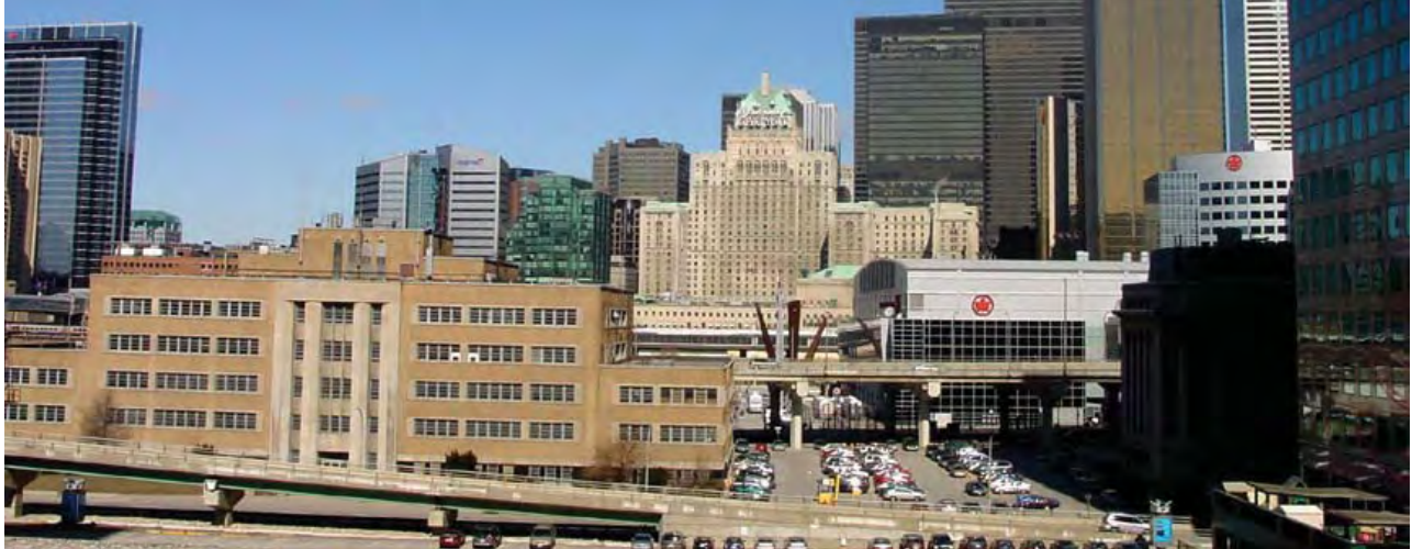
Figure 25. View of Royal York looking north from 7th floor rooftop garden, 33 Harbour Square
