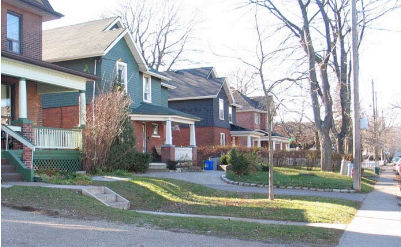
Figure 25. Looking west along Lyall Avenue, 2005.
