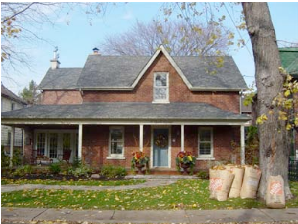
Figure 17. #74 Lyall represents typical Neo-Georgian farmhouse. This style was popular in the latter half of the nineteenth century because its second storey was “hidden”, providing a tax lower rate. While still common in rural Ontario, only a few remain in Toronto.
