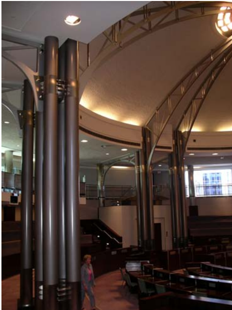
Interior view, showing the columns that support the central roof structure
