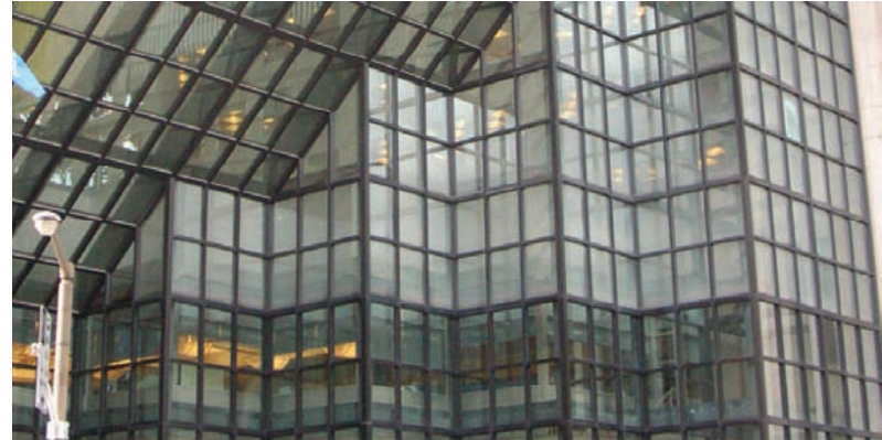
This is a good example of a design that projects sufficient visual markers for birds to perceive as a solid object. Very few dead and injured birds are found at this facade. photo credit: FLAP
