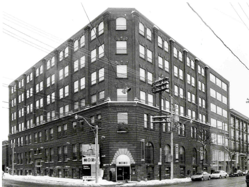
View of the south façade of the Adam Brothers Harness Manufacturing Company Building at the northeast corner of King Street East and Frederick Street.
