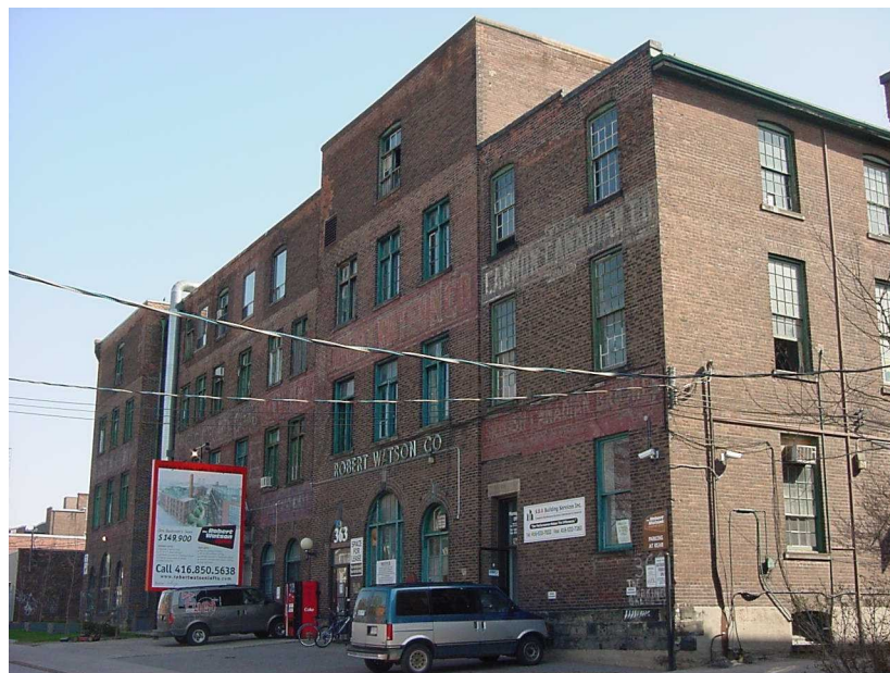
View of the principal (west) façade of the Robert Watson Factory.
