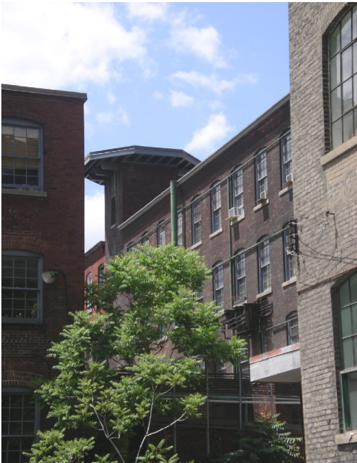
Rear (south) elevation with tower
