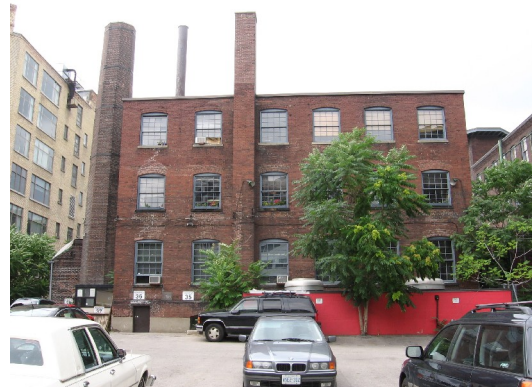
Rear (south) building with smokestack
