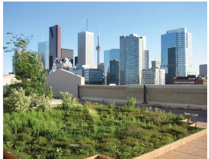
Naturalized green roofs are easy to maintain, reduce heat island effect and minimize water runoff.
