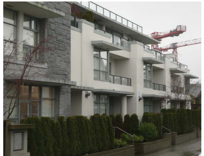
Building bases along Marine Parade should be 2-3 storeys with a 1.5 metre setback above the 3rd storey to a maximum of 4.
