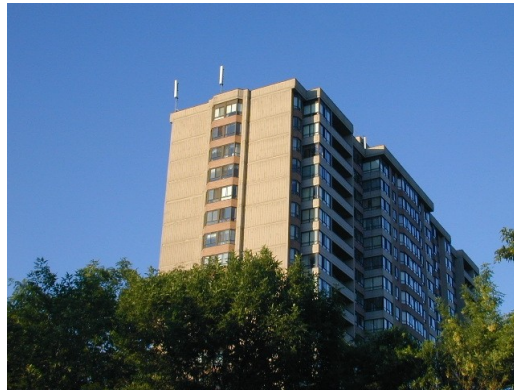
Tower on Building Roof
