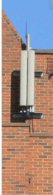
Antenna on Side of Building
