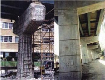
*Some corroded concrete columns have been repaired.*
