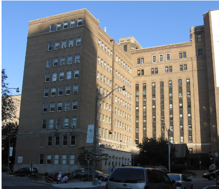
1935 hospital (centre) and 1956 south wing (left)
