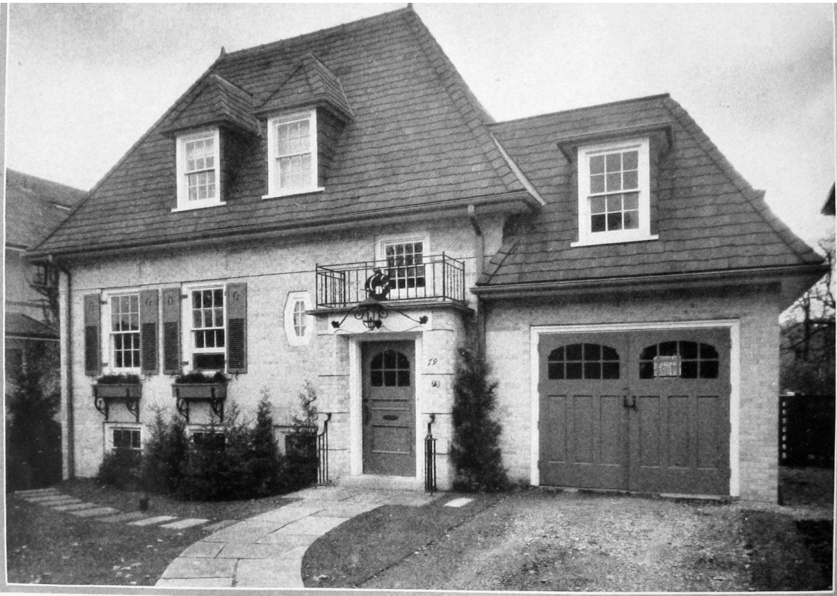
INGENUITY CREATES A HOUSE ON TWO LEVELS
