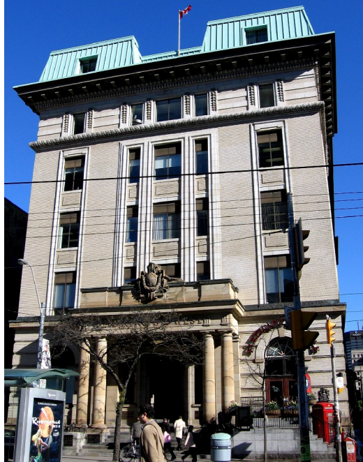
Principal (south) façade of the Union Building (the sixth floor with the mansard roof is an addition)
