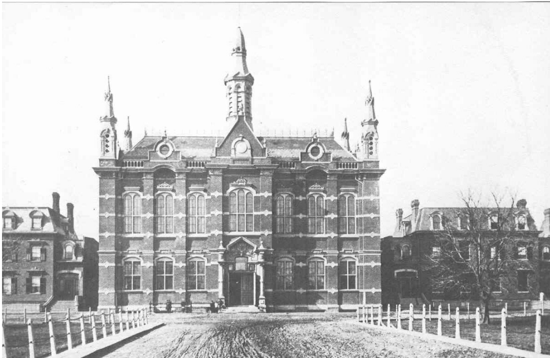
Historical photograph of Upper Canada College, showing the main campus (with the buildings facing south toward King Street West), where the Anderson Building was constructed (Source: Toronto Reference Library, Item B12-34b)
