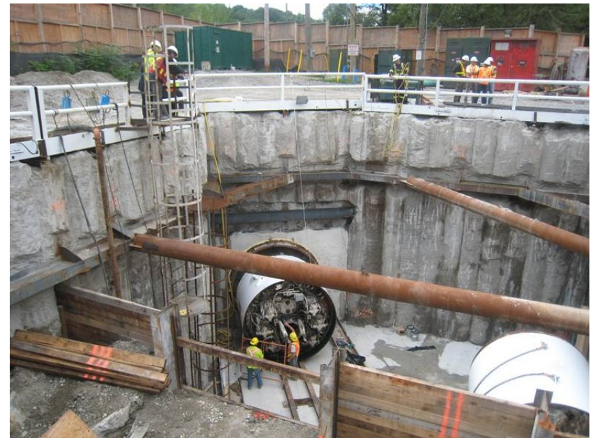
Tunnel Boring Machine-Coxwell Sanitary Trunk Sewer Bypass
