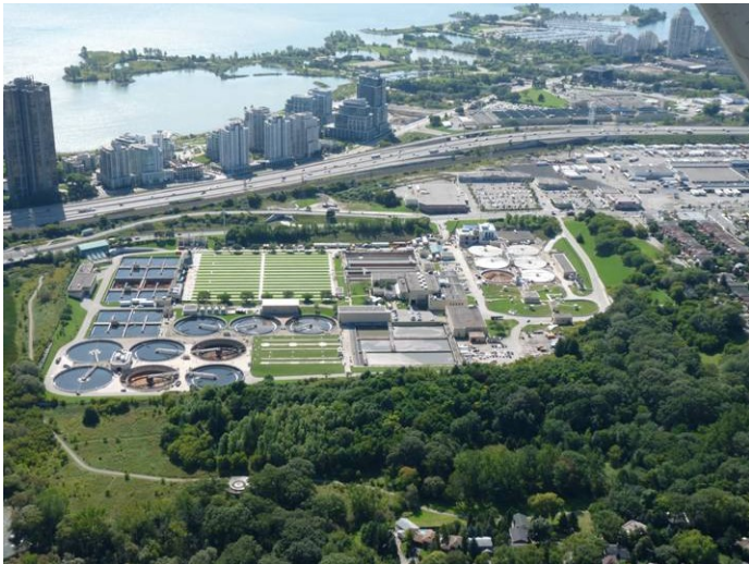
Humber Wastewater Treatment Plant
