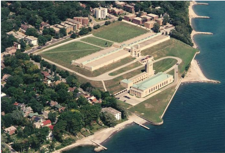
R.C. Harris Water Treatment Plant
