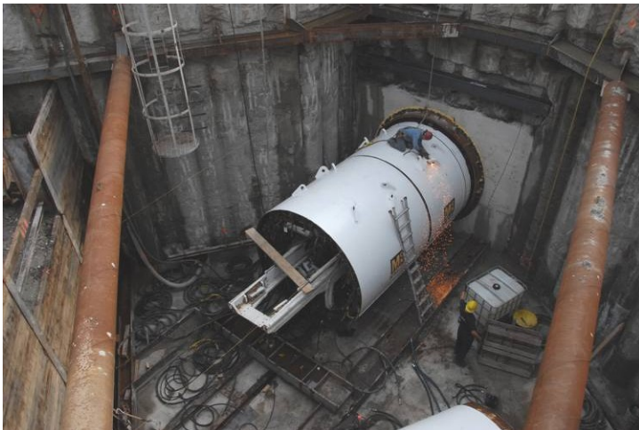
Entry Shaft-Coxwell Sanitary Trunk Sewer Bypass
