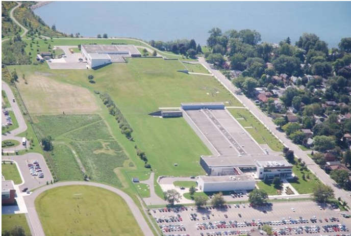
R.L. Clark Water Treatment Plant
