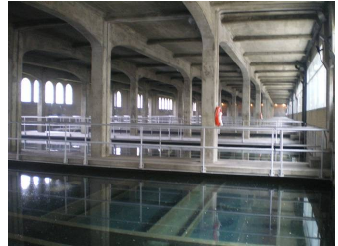
R.C. Harris Water Treatment Plant
