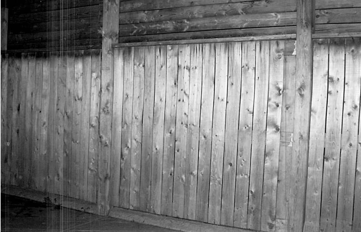
Photo # 2 – 106 Gaydon Avenue – Side Yard Fence
