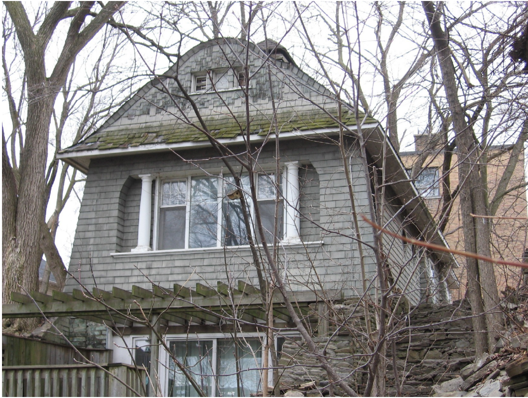
11. Photograph, Gardener's Cottage , showing the south elevation overlooking the lakefront where the lower storey is built into the side of the slope (Heritage Preservation Services, April 2011)
