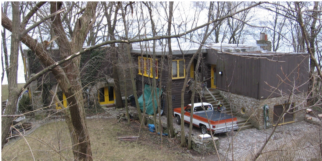
Photograph: Boathouse, Fetherstonhaugh Estate, showing the north elevation, with Lake Ontario in the background (Heritage Preservation Services, April 2011)
