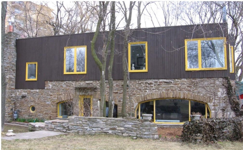
14. Photograph, Boathouse , showing the west elevation, with the tops of the former openings for boats visible in the lower storey of the wall (Heritage Preservation Services, April 2011)
