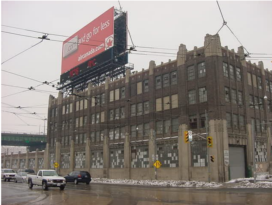
Loblaw Groceteria Building - West Elevation
