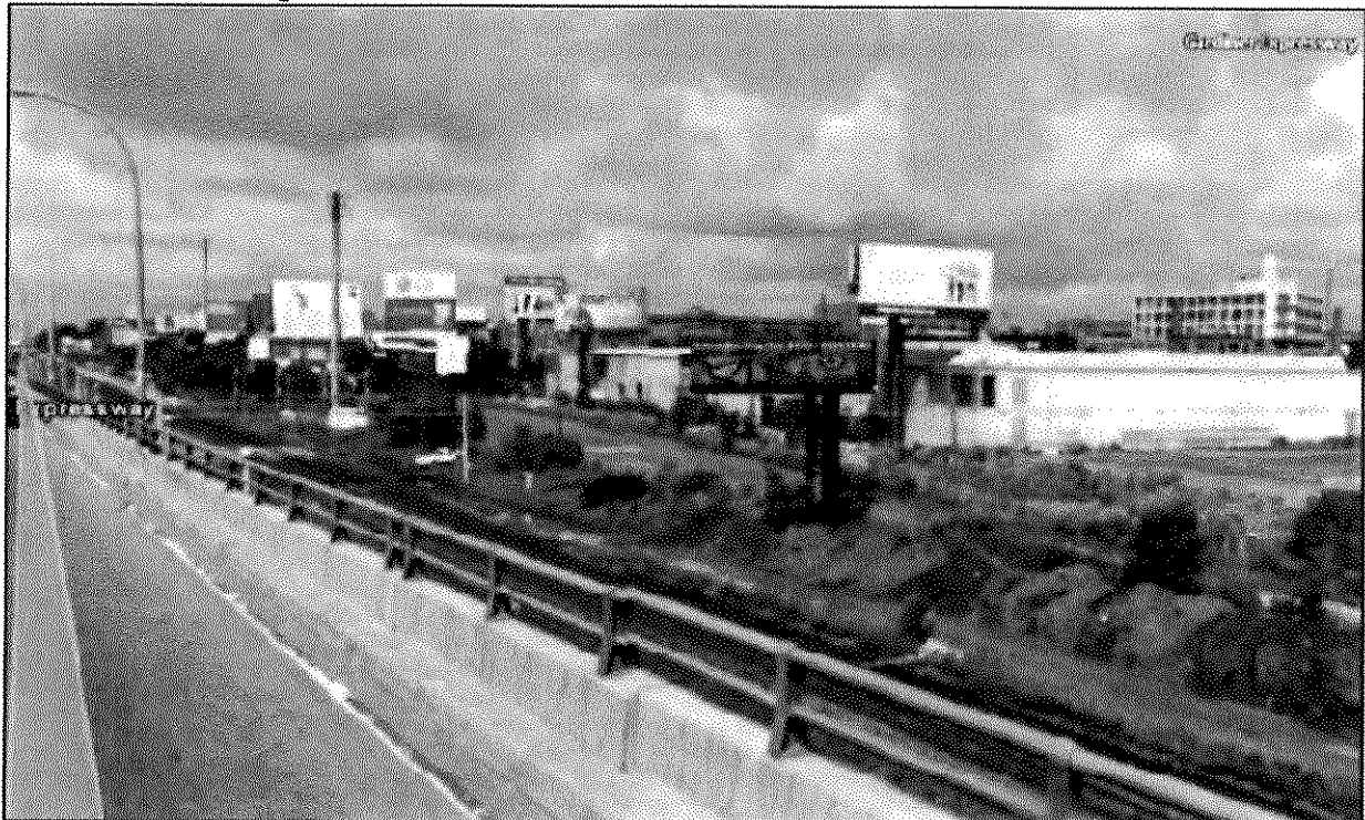
9. F.G. Gardiner Expressway; 425 metres east of Atlantic Avenue; north side; facing east
