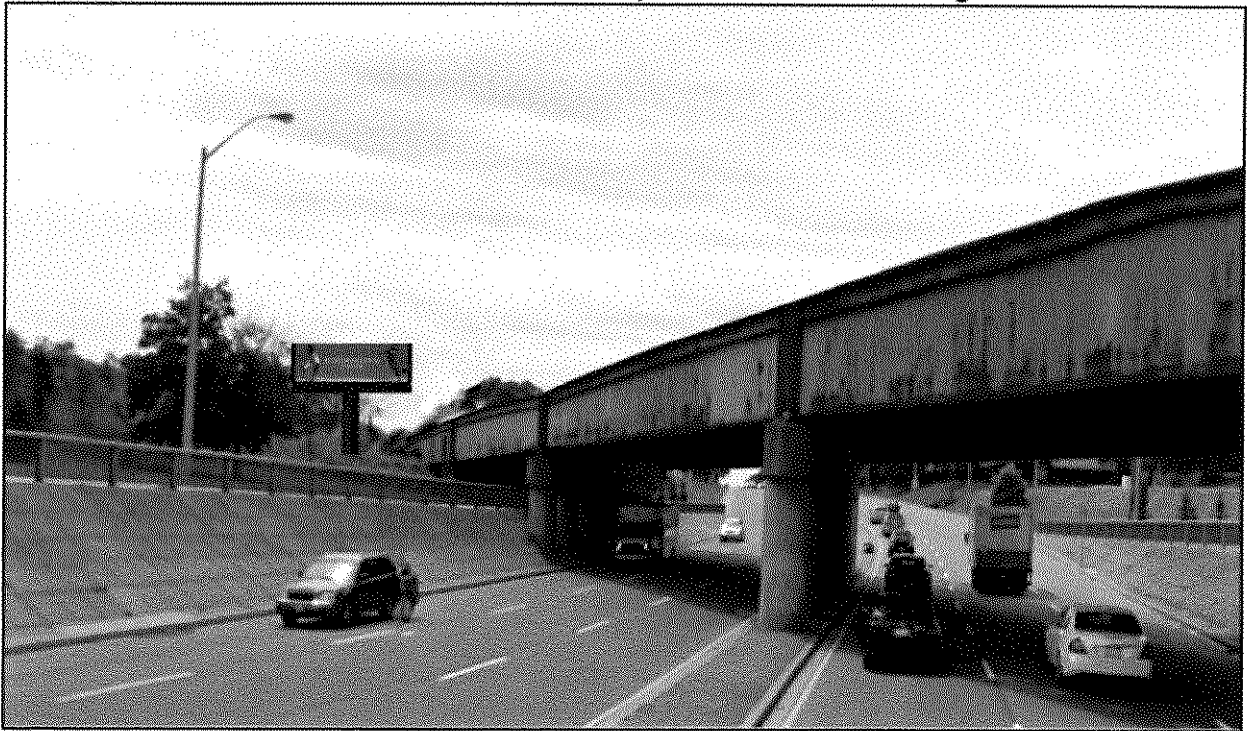
4. Leslie Street; 550 metres south of Hwy. 401; east side; facing north
