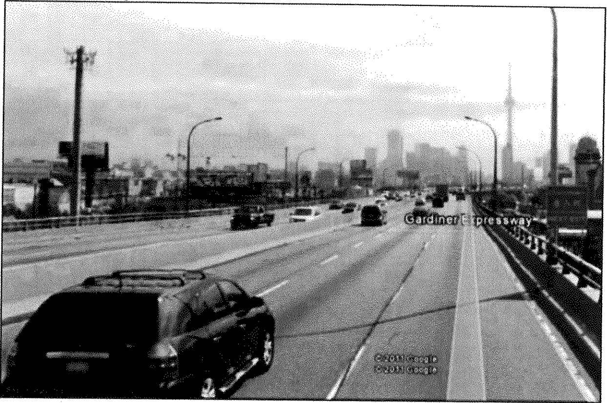
10. F.G. Gardiner Expressway; 325 metres east of Atlantic Avenue; north side; facing west
