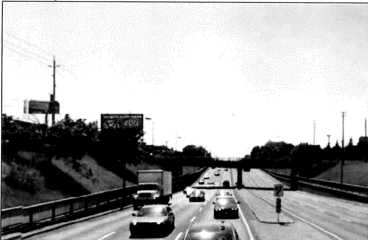
7. Steeles Avenue West; 200 metres west of Alness Street; south side; facing east
