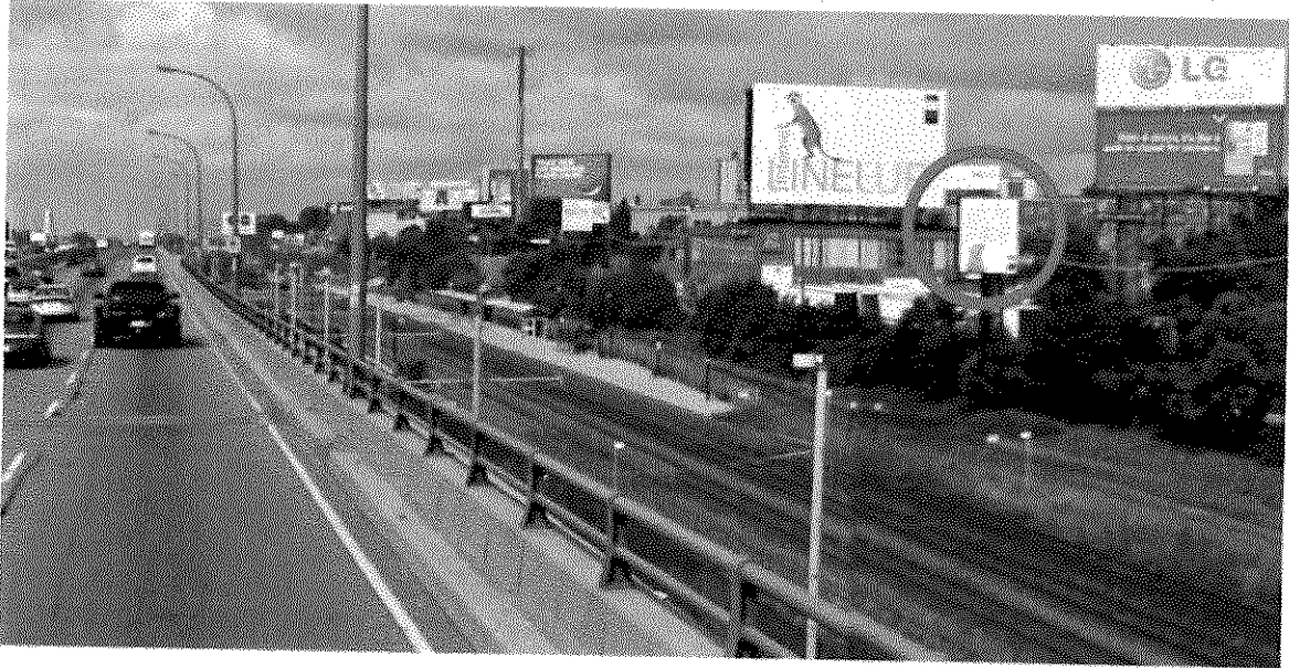
29. Gardiner Expressway; 200 metres east of Atlantic Avenue; north side; facing east
