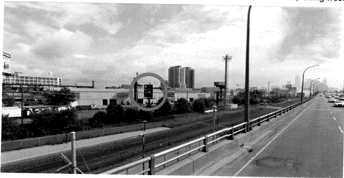
29. Gardiner Expressway; 200 metres east of Atlantic Avenue; north side; facing west
