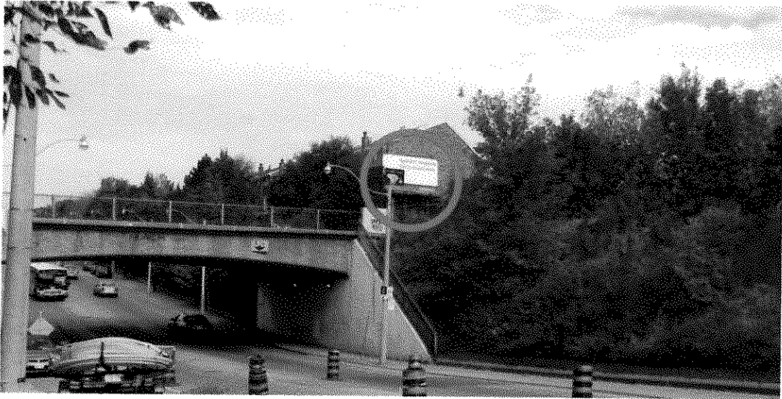
40. Greenwood Avenue; north of Walpole Avenue; east side; facing south
