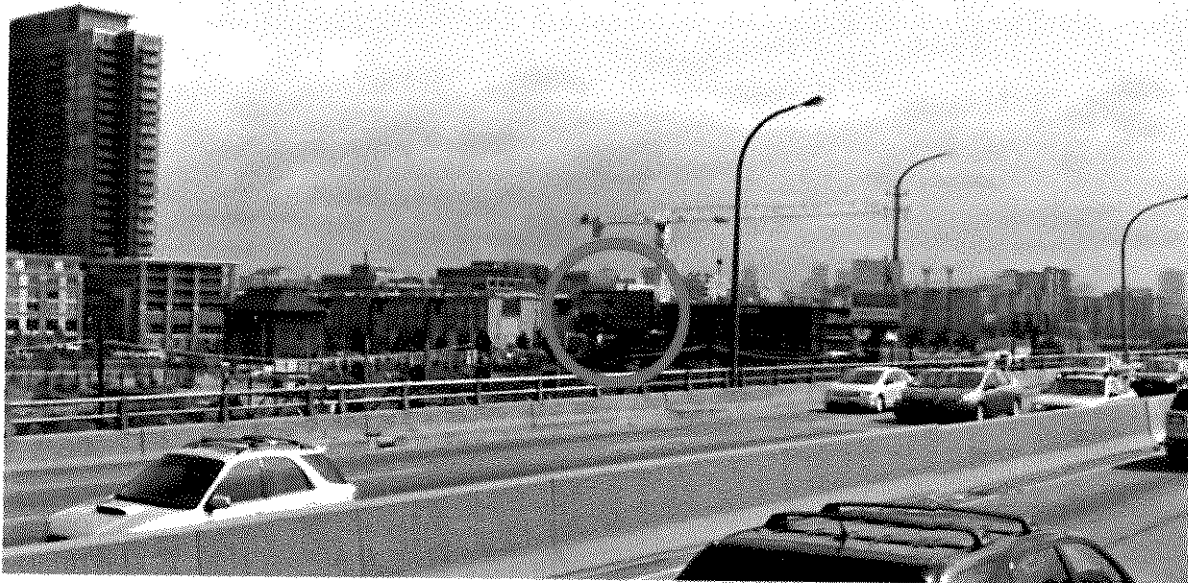
33. Gardiner Expressway; 425 metres east of Atlantic Avenue; north side; facing west
