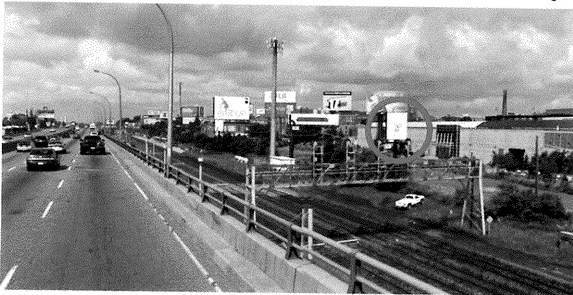
37. Gardiner Expressway; 325 metres east of Atlantic Avenue; north side; facing east
