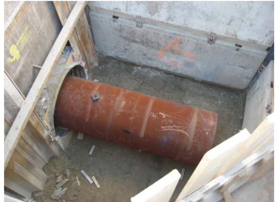
Steel welded pipe (1650 mm used for Neilson Road project)
