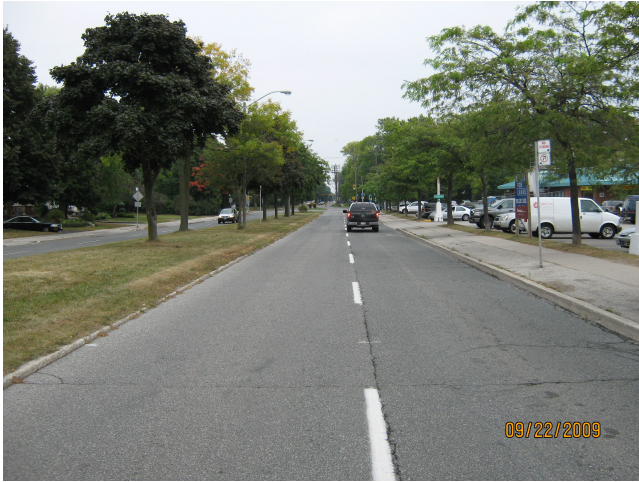
Eastbound view south of the plaza driveway on the South side
