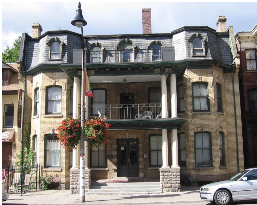
Principal (east) façade
