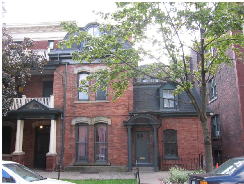
North elevation on Gloucester Street
