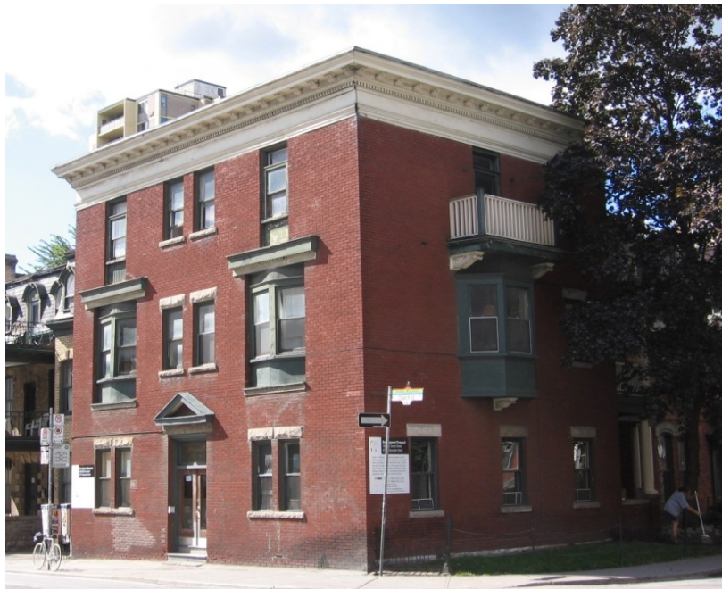
East façade on Church Street (left) and north elevation on Gloucester Street (right)
