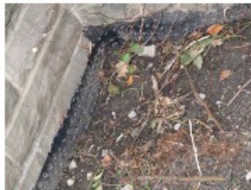
Fig 17. Damp proof layer on west foundation. (ERA)
