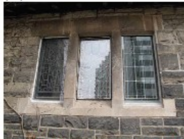
Fig 26. Exterior storms on casement windows. (ERA)
