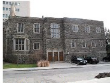
Fig 12. West elevation, rear. (ERA)
