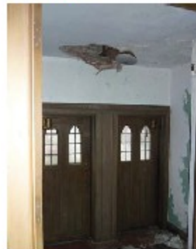
Fig 45. West tower entrance. (ERA)
