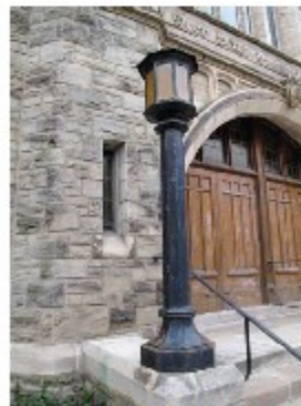
Fig 34. Light standard at main entrance. (ERA)
