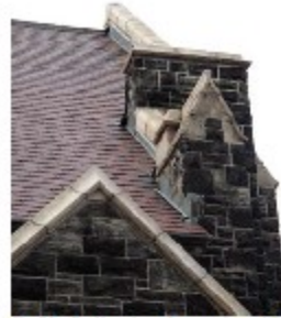
Fig 21. Spall and mortar repair on NE buttress cap. (ERA)
