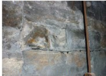
Fig 36. Damp proof layer in foundations. (ERA)
