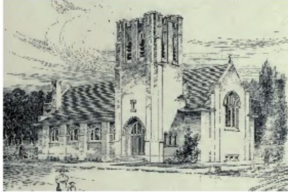
Fig 15. St Barnabas Anglican Church, Sharp & Brown Architects, 1910. (Construction)
