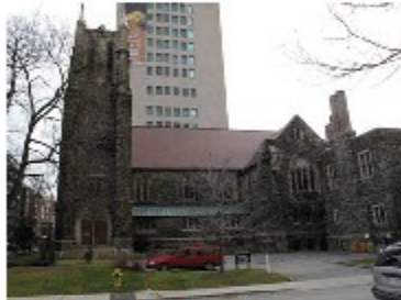
Fig 11. West elevation, front. (ERA)
