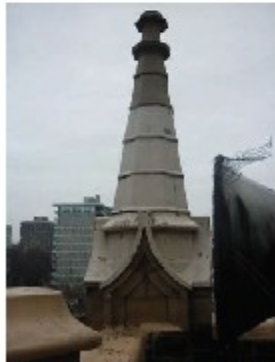
Fig 50. Painted coating on tower finial. (ERA)
