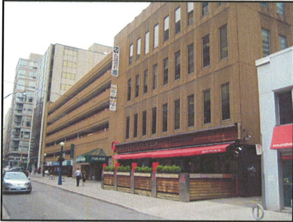
South side of subject, looking north west
