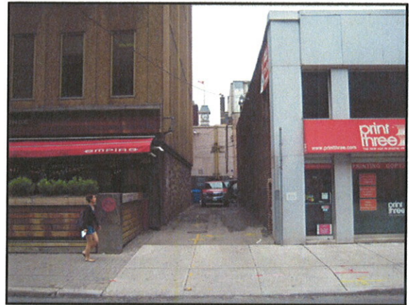
Eastern limit of the subject property
