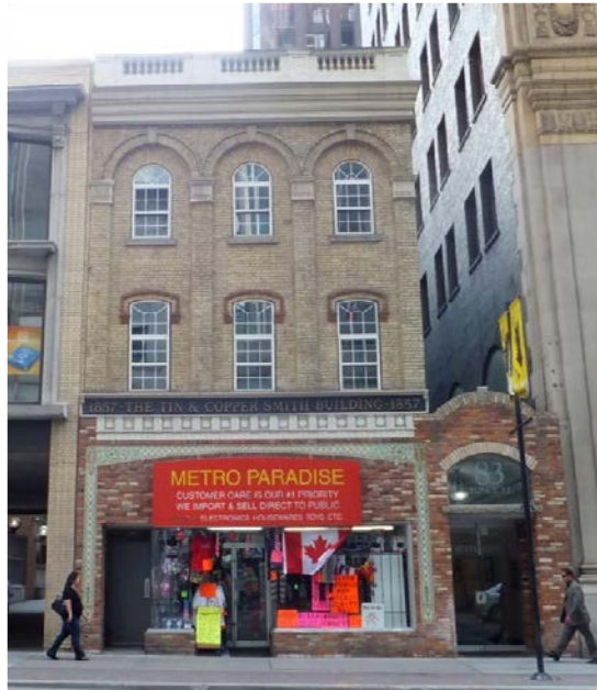
28. Photographs, Low-Rise Heritage Buildings on Yonge Street between Front and Queen Streets, June 2012: on the east side, north of King Street, the Piper Building (1857) at 83 Yonge Street (Heritage Preservation Services)
