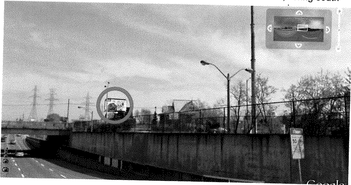
4. Kipling Avenue; 175 metres north of Belfield Road; east side; facing south
