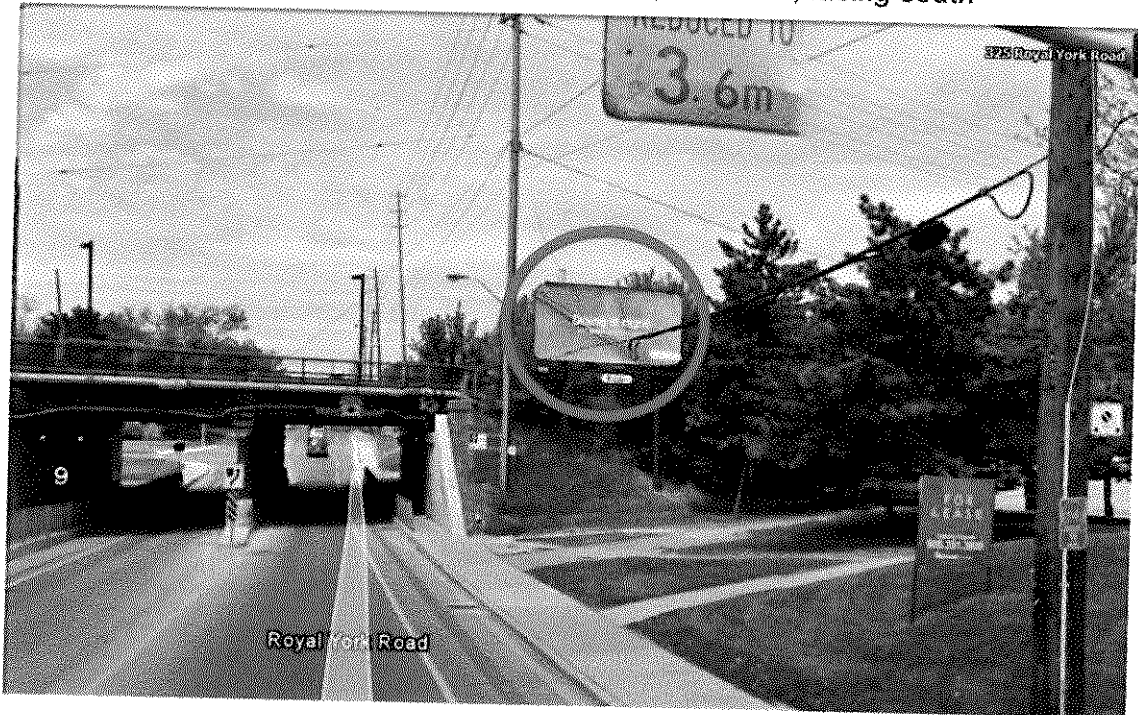
7. Royal York Road; north of Cavell Avenue; east side; facing south
