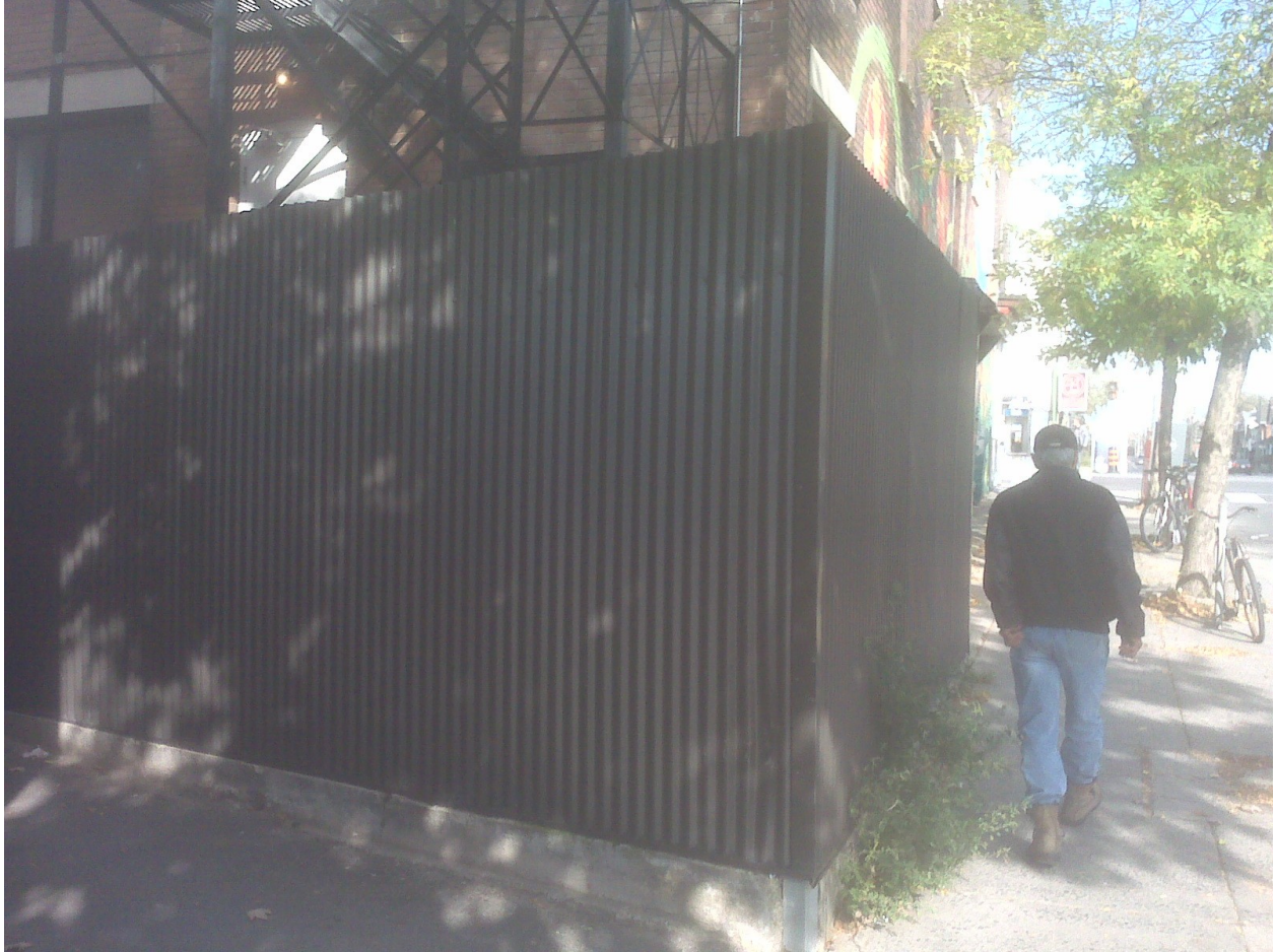
Attachment 1 – 1485 Dundas Street West - photograph of fence on east and south sides of property
