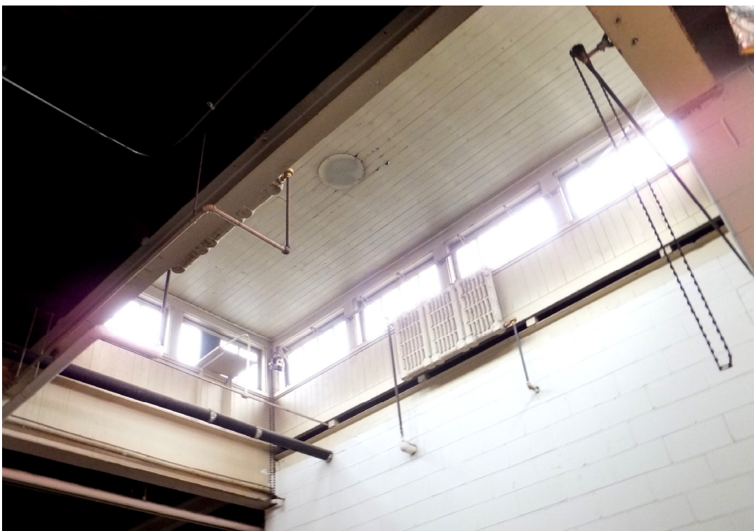
25. Photographs, Waterworks Building : showing the exterior and interior views of one of the wood monitors with exterior metal detailing that are positioned above the workshops (Heritage Preservation Services, January 2012)
