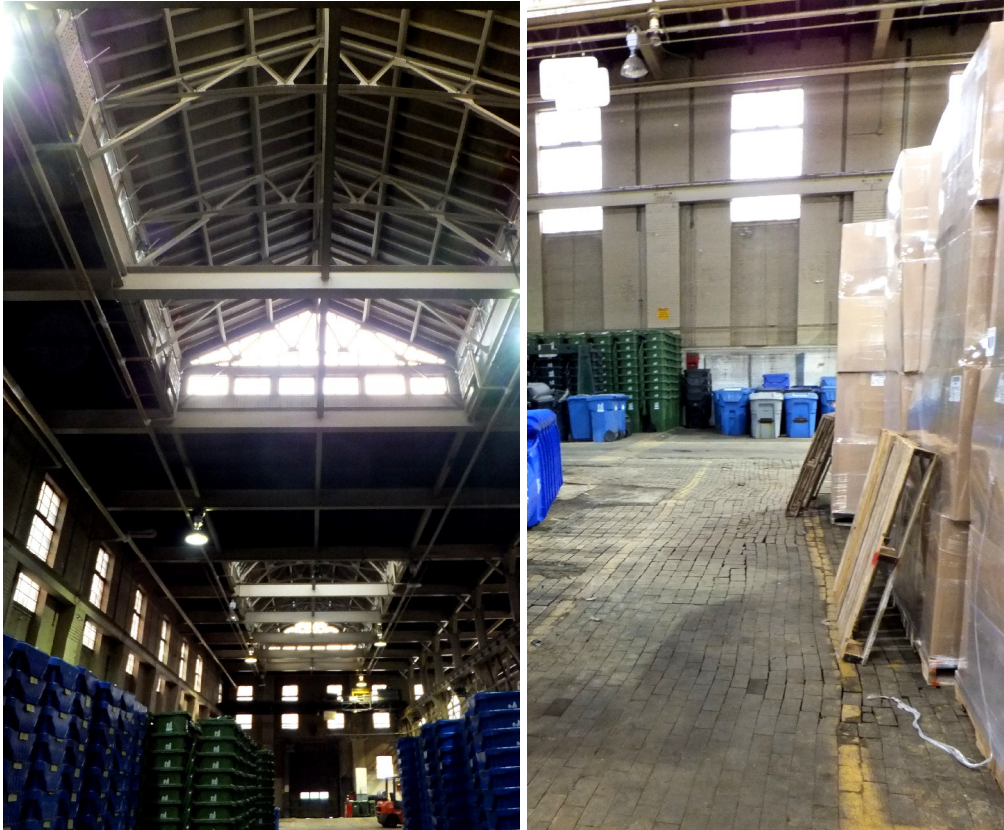
26. Photographs, Waterworks Building : showing the interior of the warehouse and workshops with one of the metal truss skylights (left) and the wood floor (right) (Heritage Preservation Services, January 2012)
