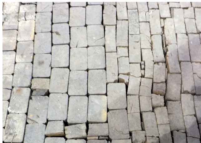
27. Photograph, Waterworks Building : showing a detailed view of the rare wood floor in the workshops where pieces of wood are laid in a pattern mimicking masonry (Heritage Preservation Services, January 2012)
