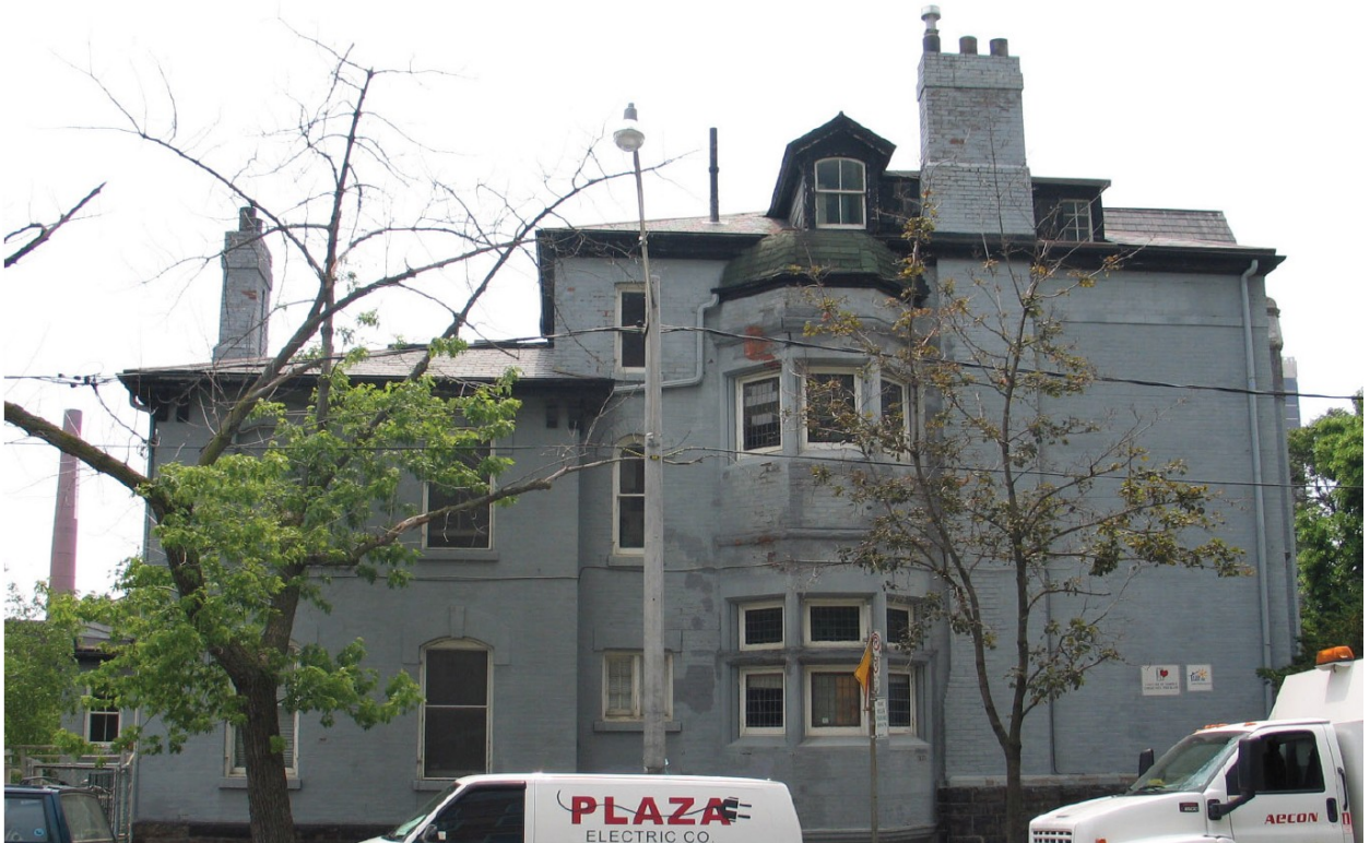
Alteration of a Heritage Property – 571 Jarvis Street / 119 Isabella Street (Casey House Hospice)
