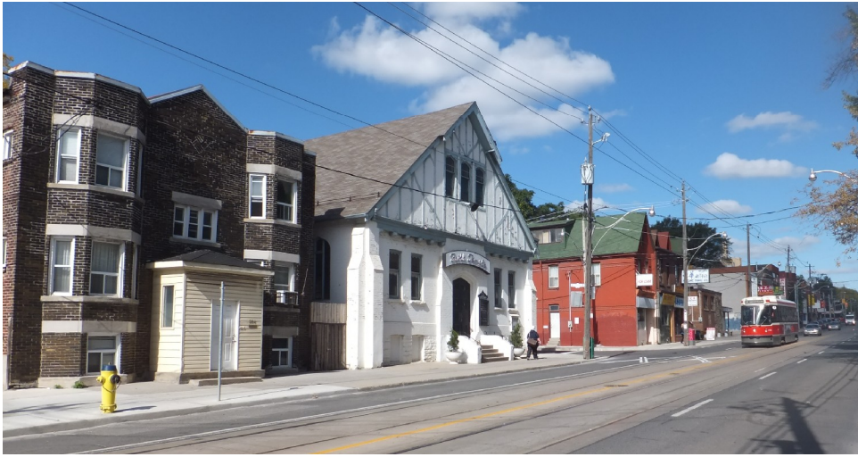
13. Current Photograph, September 2012: view looking north along the west side of Broadview Avenue to the church on the southwest corner of Mount Stephen Street (Heritage Preservation Services)
