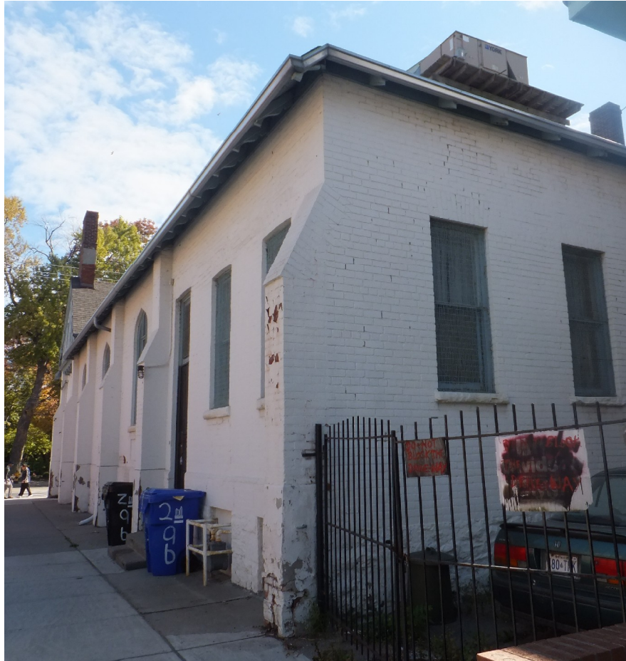
11. Current Photograph, September 2012 : showing the east elevation flanking Mount Stephen Street on the left with the rear (west) wall on the right (Heritage Preservation Services)
