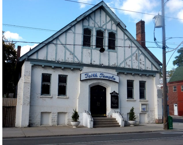
Principal (east) façade of Broadview Avenue Congregational Church (Heritage Preservation Services, September 2012)
