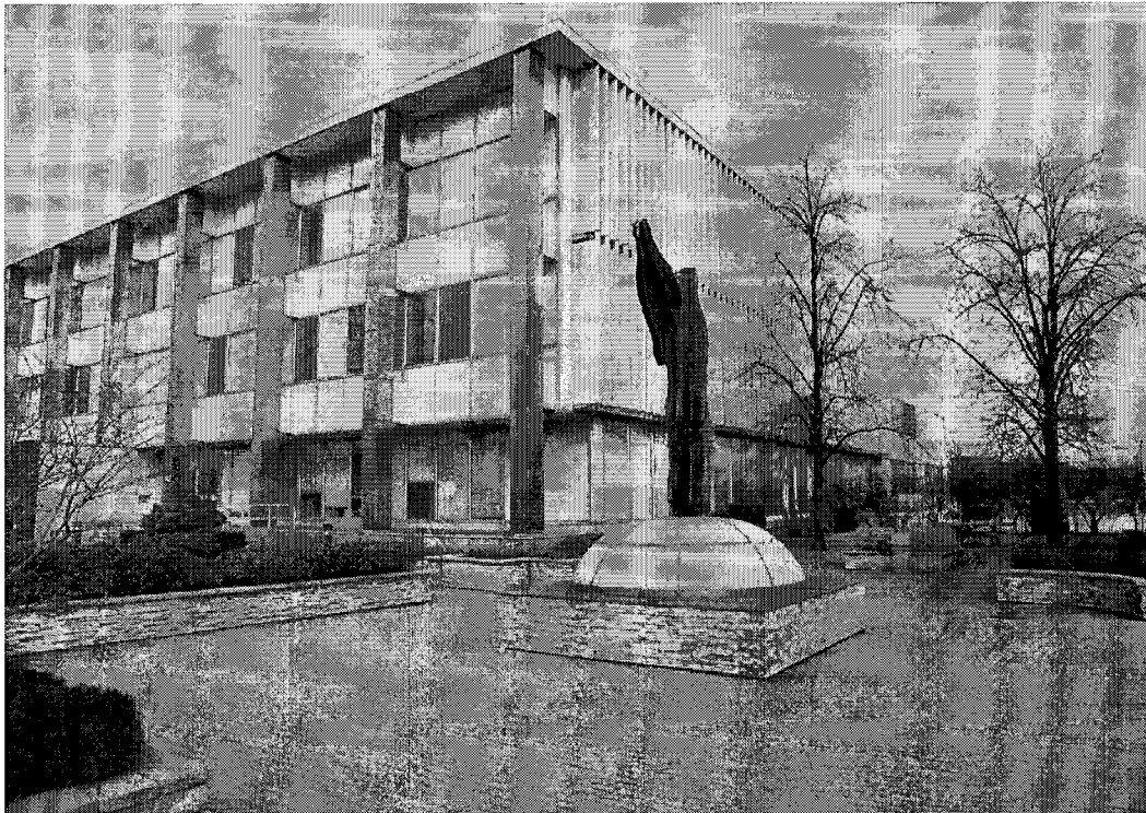
Above: principal (south) façade of the Coca-Cola Office Building Below: "Coca-Cola" sculpture in the courtyard adjoining the office building (left) (Heritage Preservation Services, March 2013)
