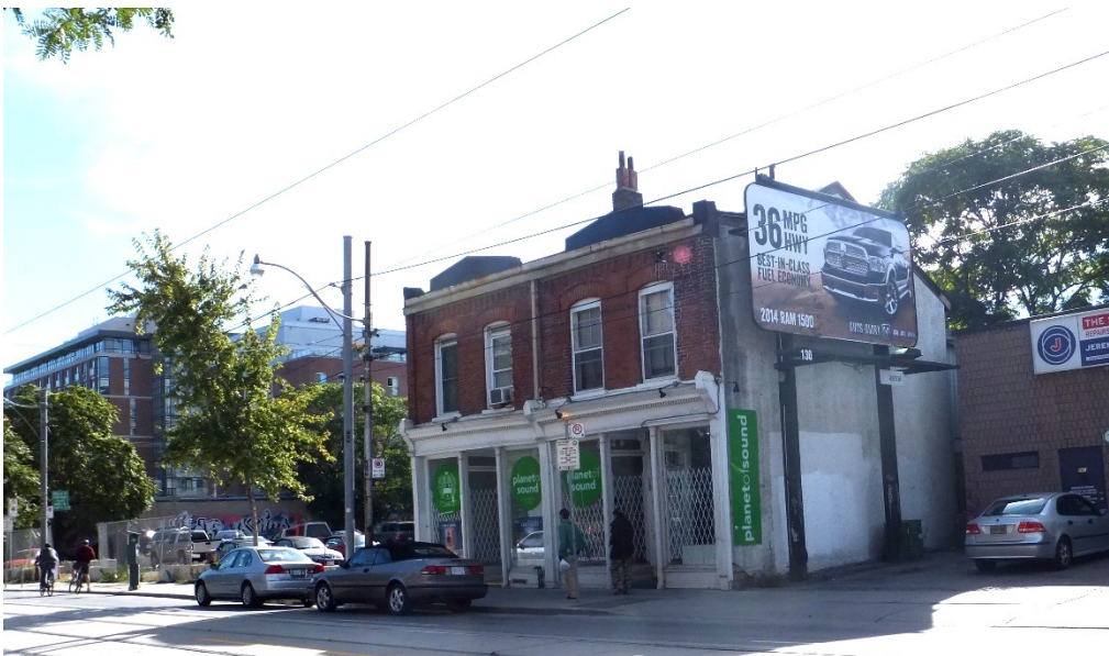
Showing the principal (north) façades (above) and the context of the Christina Lauder Buildings on Queen Street East (below) (Heritage Preservation Services, September 2013)
