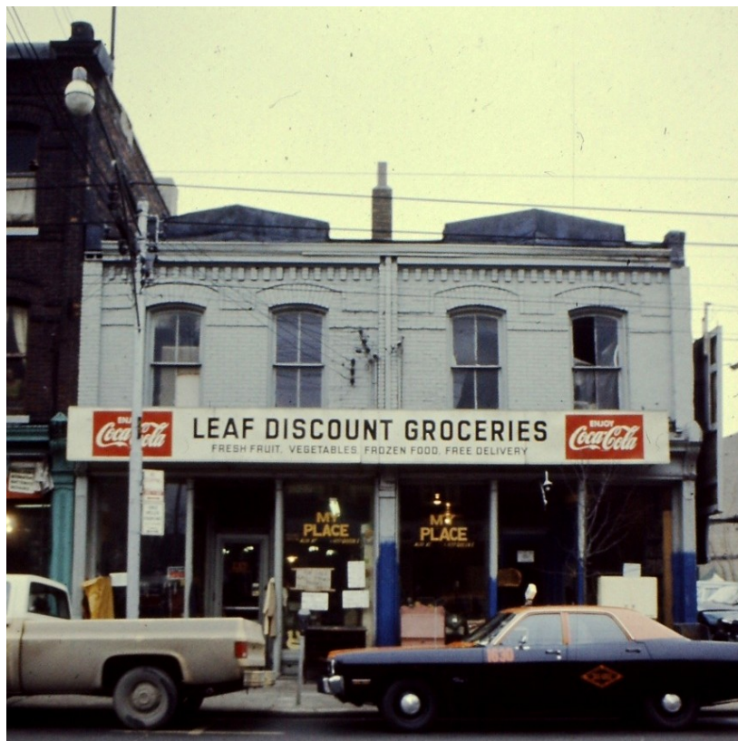
10. Archival Photograph, 263-265 Queen Street East, c.1973 : showing the buildings with the brickwork painted (Toronto Historical Board)
