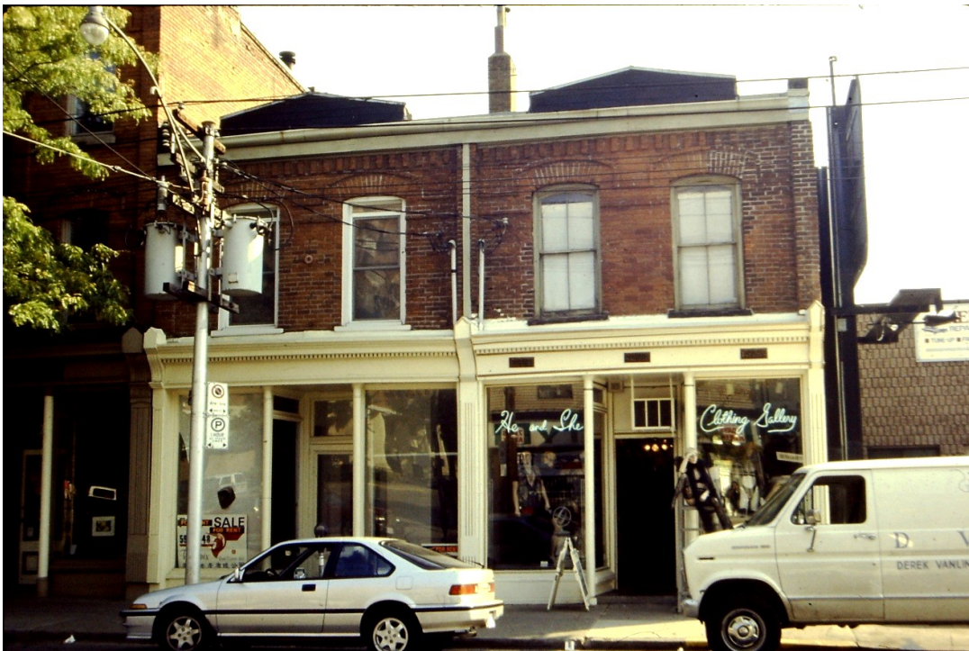
12. Archival Photograph, 263-265 Queen Street East, 1993: showing the storefronts with recessed entrances and the decorative brickwork on the second-storey openings and beneath the roofline (Toronto Historical Board)
