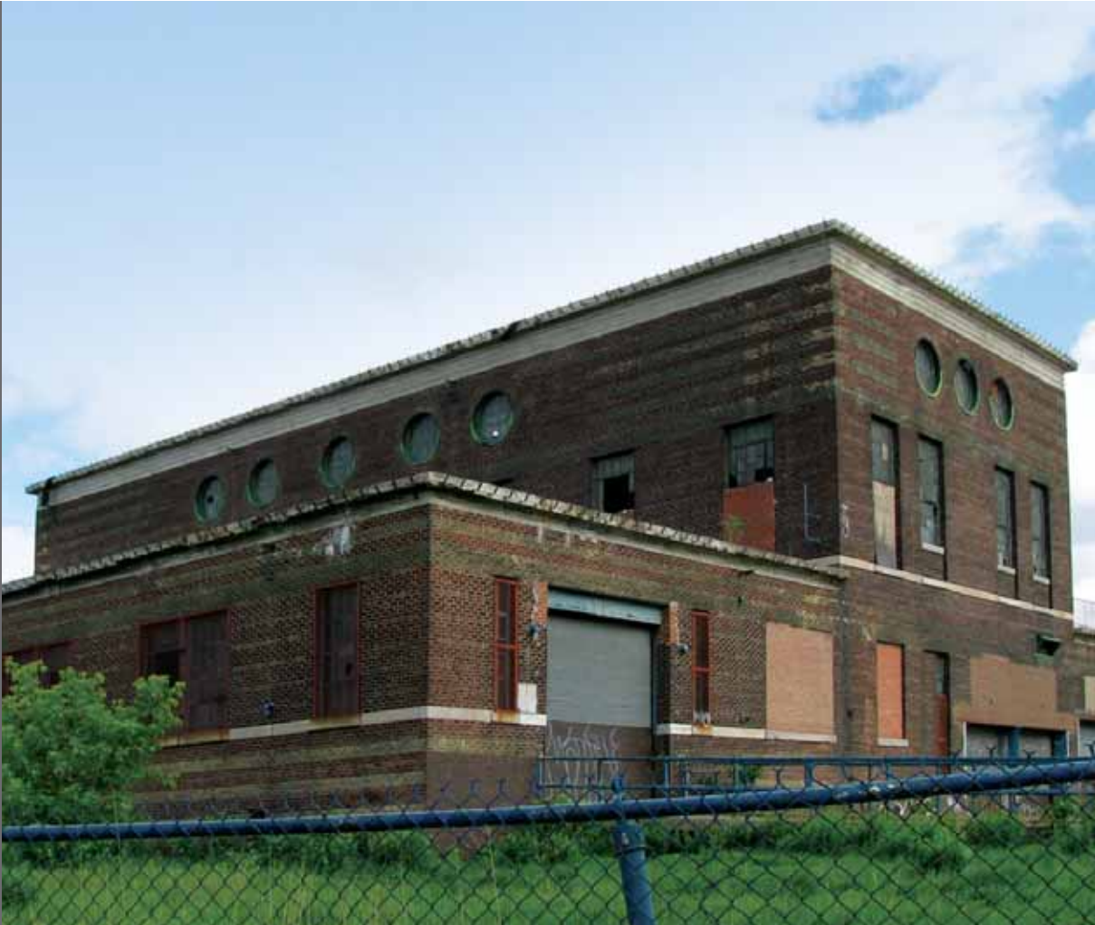
150 SYMES ROAD Heritage designated industrial building.
