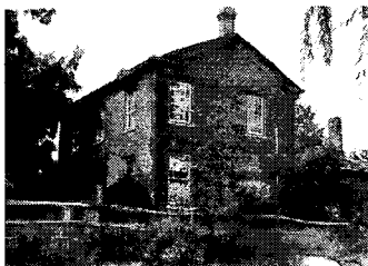
72 OLD BURNHAMTHORPE RD. SAMUEL & ANN MERCER FARM Built ca. 1820-30
