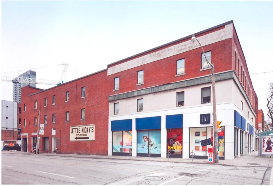
North east corner of site (looking west)
