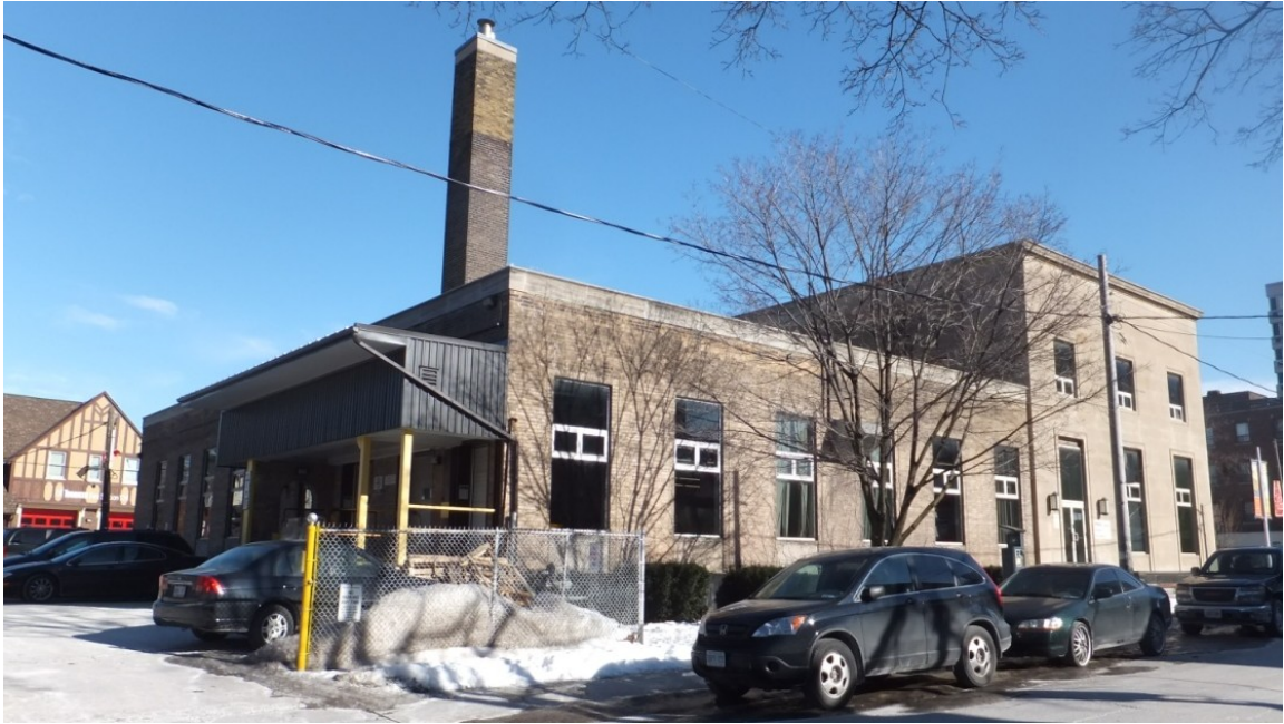
25. Photograph, 2384 Yonge Street, 2013 : showing the south elevation on Helendale Avenue on the right and the rear (west) wall to the left (Heritage Preservation Services)
