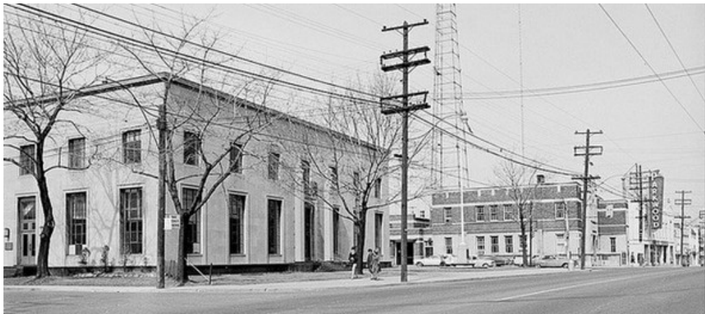
20. Archival Photograph, Yonge Street and Montgomery Avenue, 1968 : showing the placement and setback of Postal Station “K” on the southwest corner of the intersection and Police Station #12 to the north (City of Toronto Archives, Series 648, Item 18)
